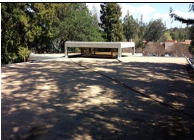
I Police Headquarters Roof Repair
