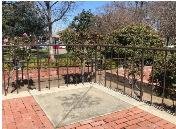
H Plaza Level Railings – Code Upgrade
