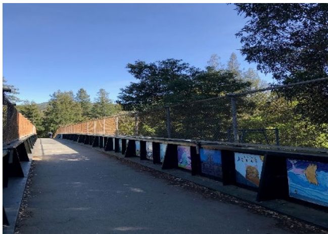
E Forbes Mill Footbridge Improvements
