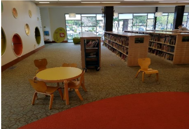
G Library Carpet Replacement
