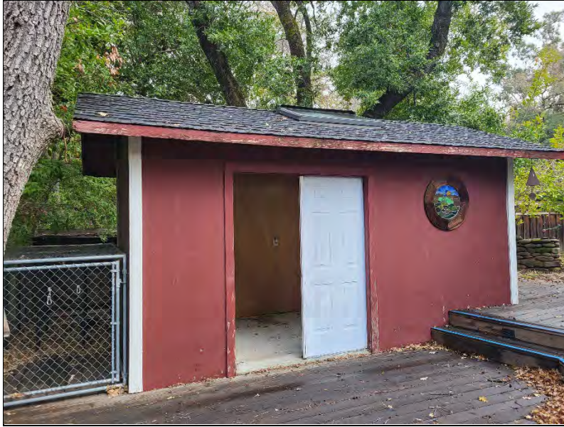
Figure 8. 32 Euclid Avenue Shed (view north/northwest; January 10, 2023).
