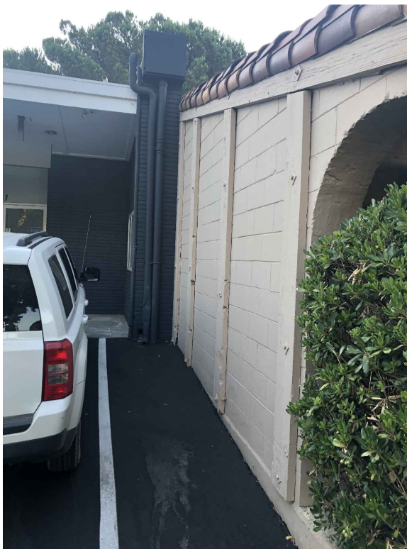
Photo of Side of Existing Building
