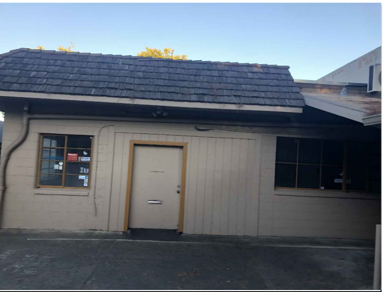
Photo of Rear of Existing Building
