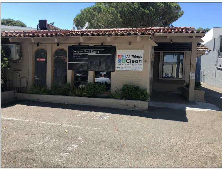
Photo of Front of Existing Building
