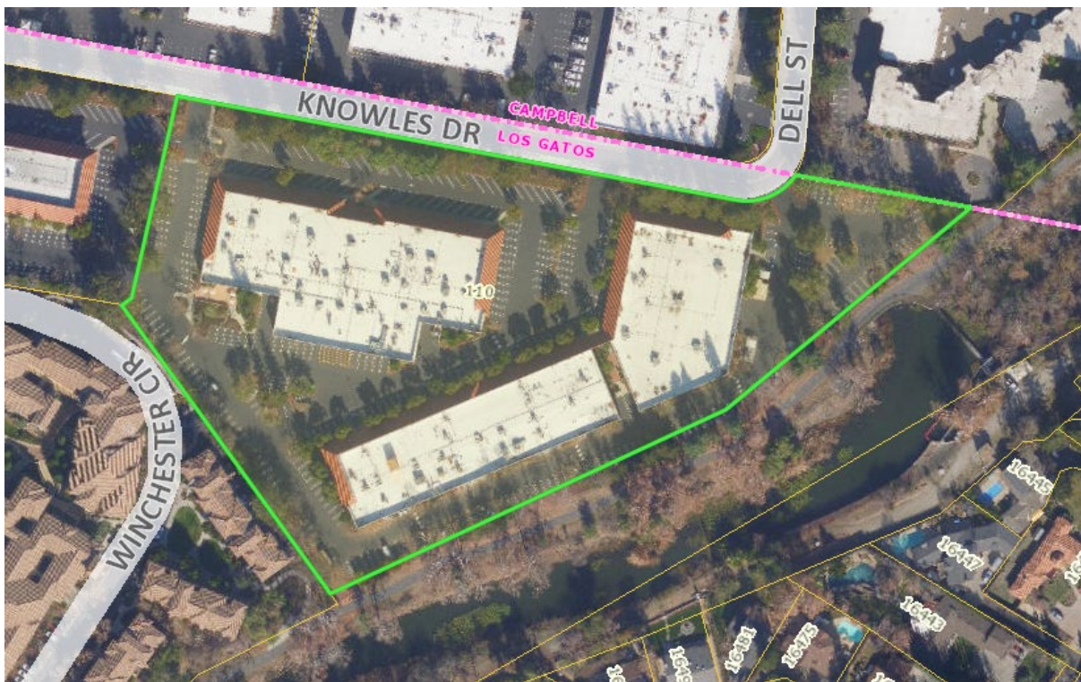
Figure D-30 Knowles Drive (Site F-1)
