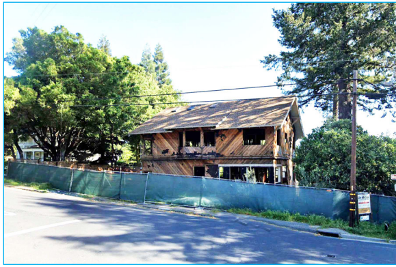
The Site and former structure facing Hernandez Avenue
