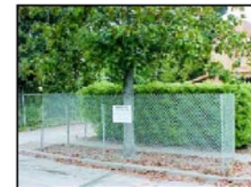
IMAGE 2.15-3 Tree Protection Within a Planter Strip
