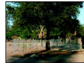
IMAGE 2.15-2 Tree Protection Fence at the Dripline
