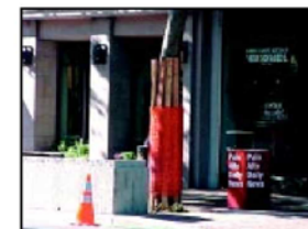
IMAGE 2.15-4 Trunk Wrap Protection
