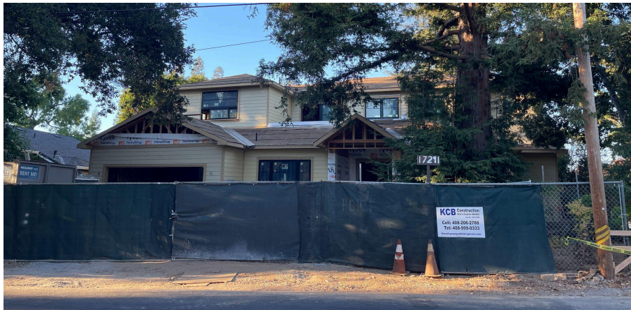
Front Facade of 17291 Wedgewood Ave (Under Construction)
