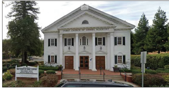
2 FIRST CHURCH OF CHRIST SCIENTIST (BUILDING HEIGHT: ±29) 238 E MAIN ST, LOS GATOS, CA 95030
