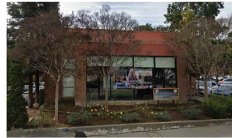
208 E MAIN STREET ( BUILDING HEIGHT ±18')
