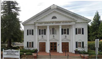
238 E MAIN STREET (BUILDING HEIGHT ± 29')
