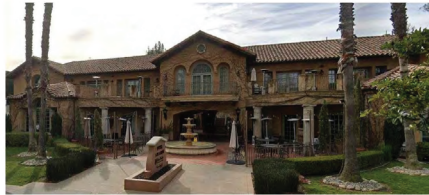
210 E MAIN STREET (BUILDING HEIGHT ±30')
