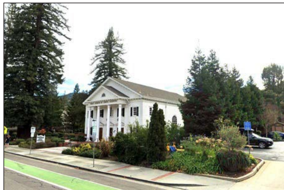
Nearby church across East Main Street
