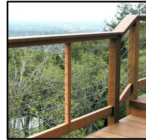
GUARD RAIL AT POOL AREA
