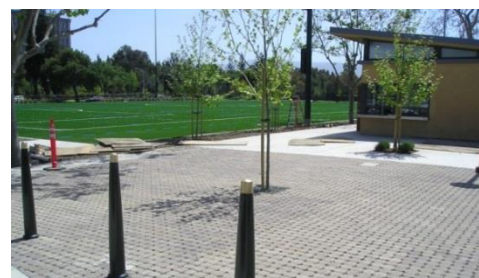
Figure 2-3 Permeable Pavers, Mayfield Playing Fields, Palo Alto (Source: City of Palo Alto)
