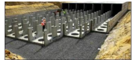
Figure 2-8 Subsurface vault for rainwater harvesting, under construction (Source: Conteches.com)
