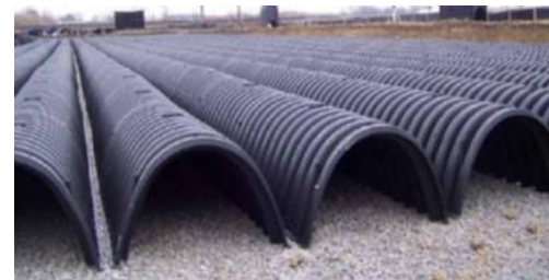
Figure 2-5 Subsurface infiltration system, (Source: Conteches.com)
