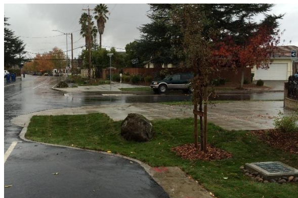
Figure 2-1 Stormwater curb extension, Hacienda Avenue, Campbell (Source: City of Campbell)
