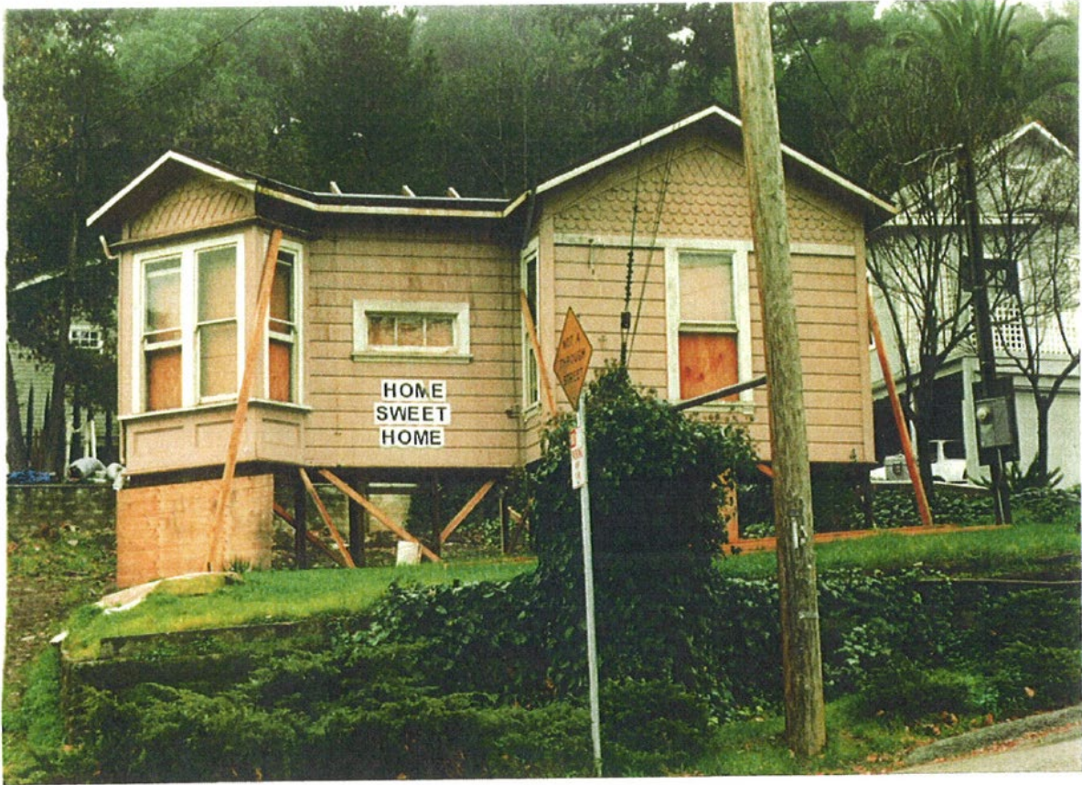
REBUILDING HOUSE AT 93 BROADWAY
