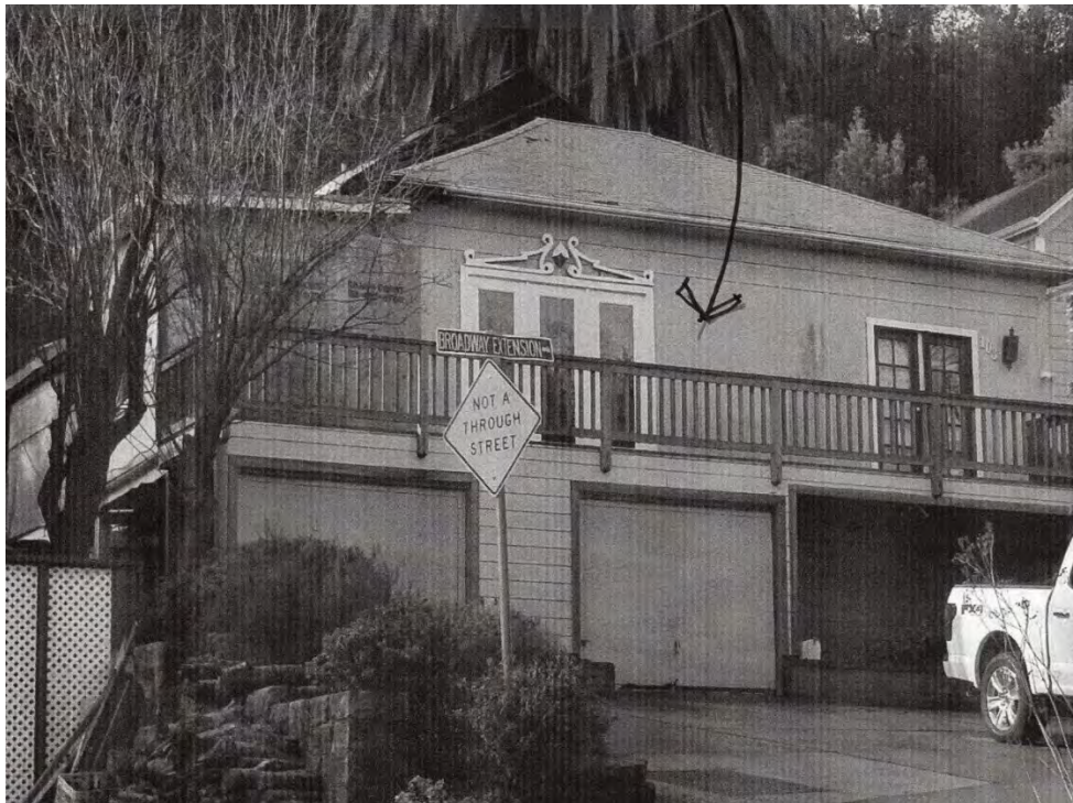
Exhibit A – The existing structure
