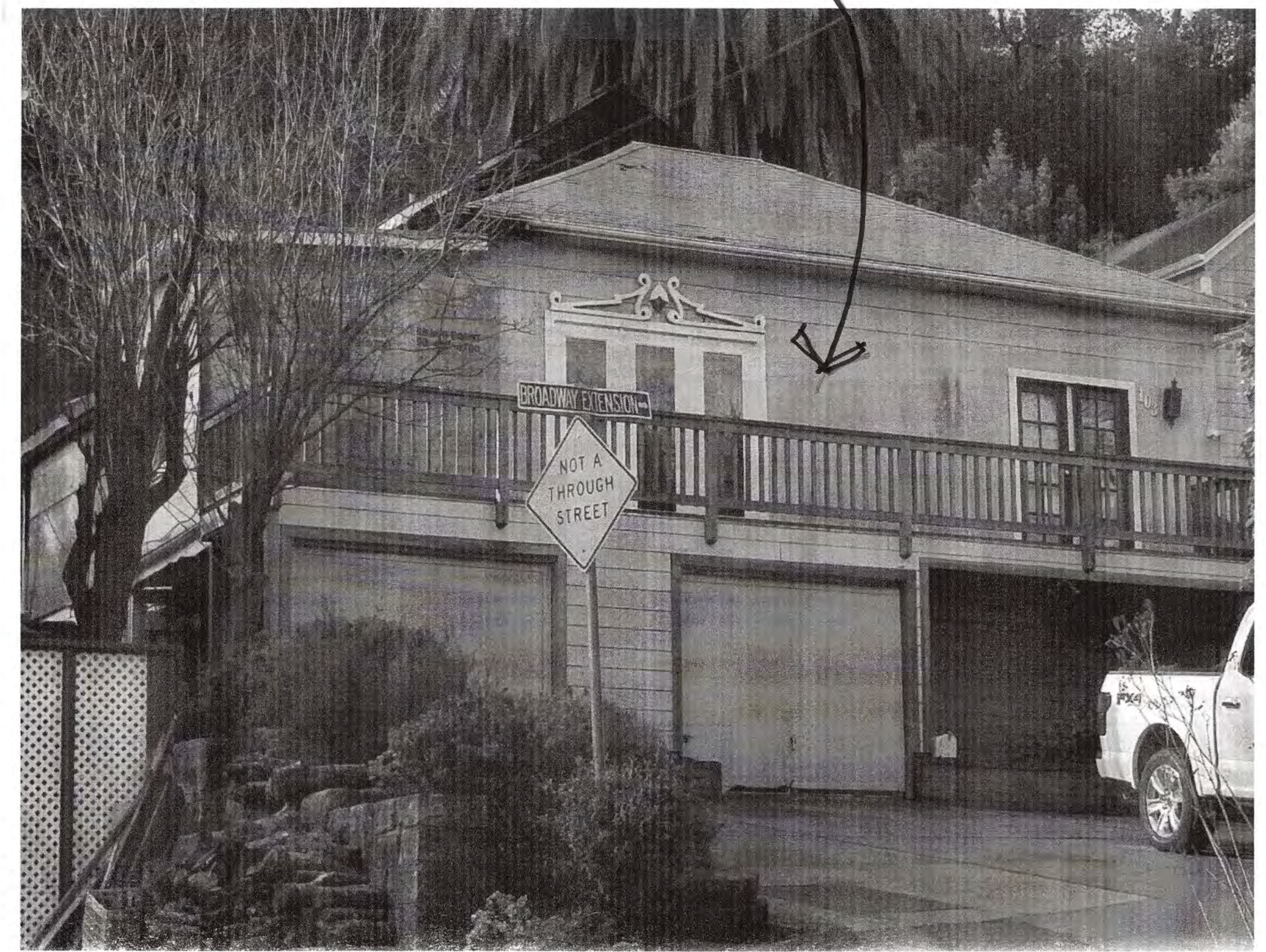
PHOTO OF EXISTING STRUCTURE.
