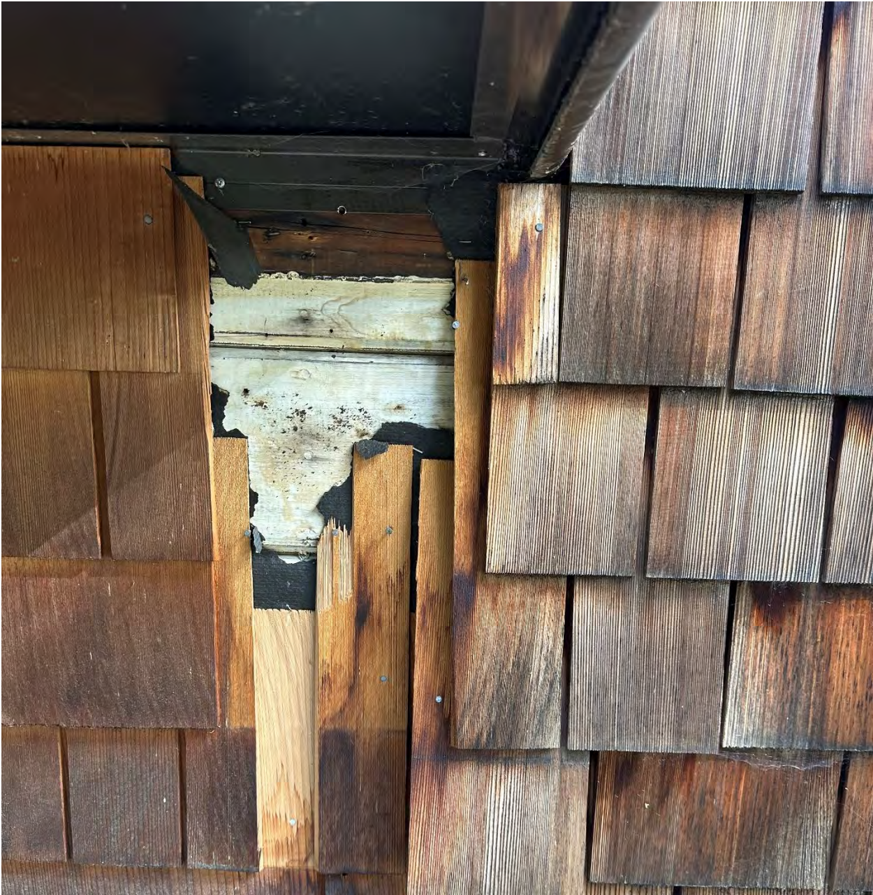
#6: South Side – Middle (original siding):
