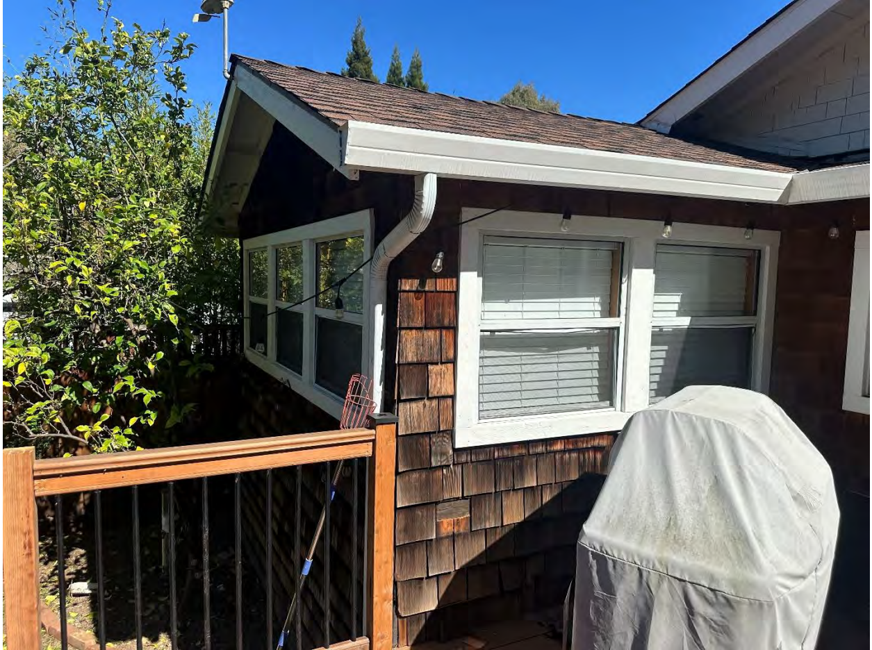
Rear Side post-1956 Constructions
