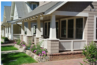
Porch columns, bases, caps, beams and railings
