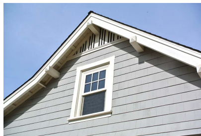
Gable end beam ends and vent detail
