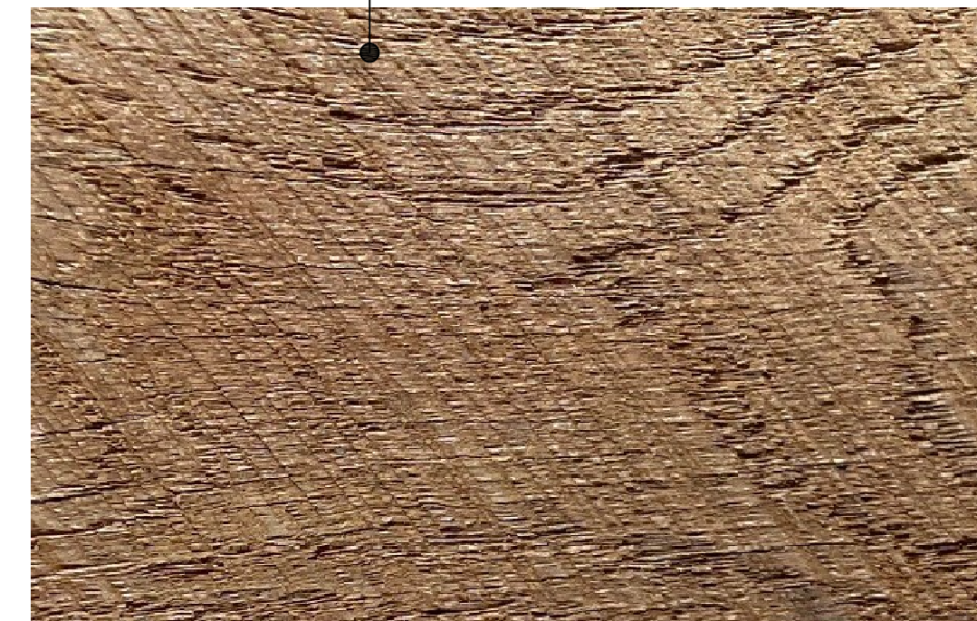
WOOD SHINGLE ROOF
