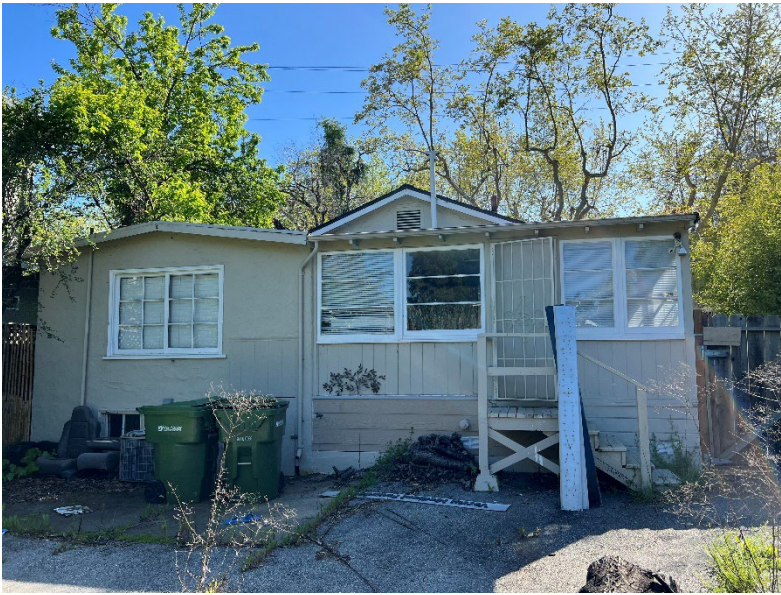
Photograph 4 – Rear elevation Looking southwest Infill addition on the right. Owner's photo 2024
