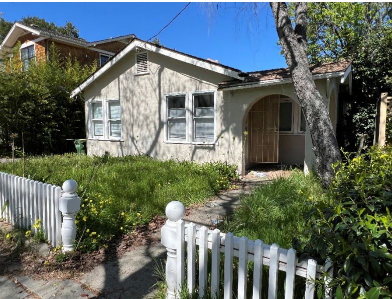
Photograph 5 – Street façade Owner's photo 2024 with fence; Looking north
