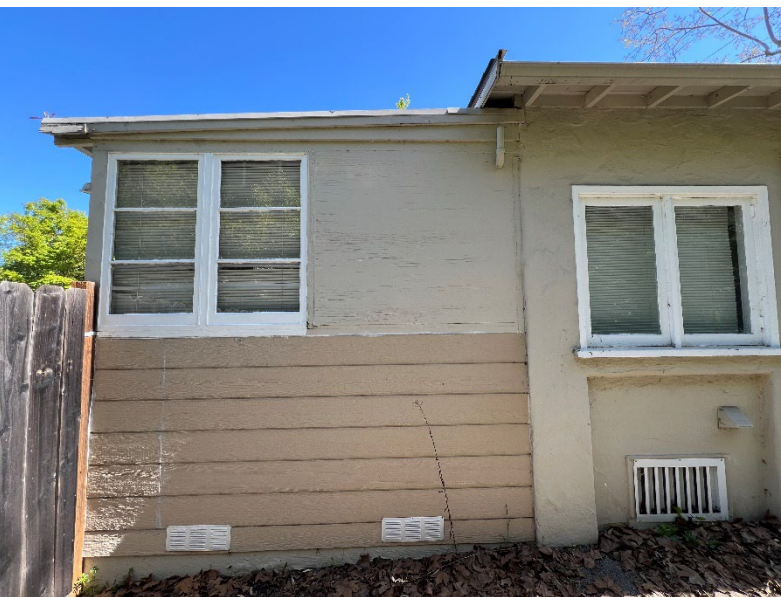
Photograph 6 – Northwest side detail; Looking southwest. North corner infill addition. Owner's photo 2024
