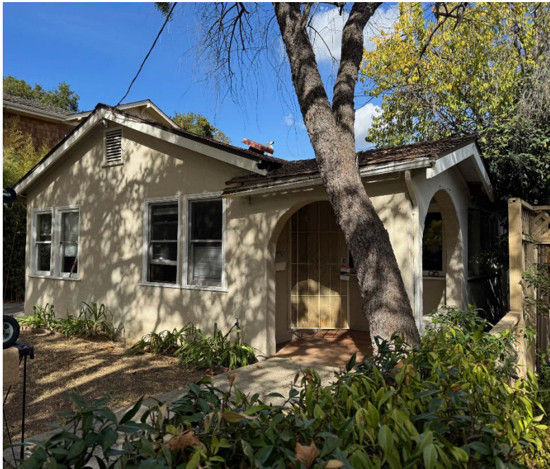
Photograph 3 – Street façade and south corner Looking north. MBA photo 31 OCT 2024
