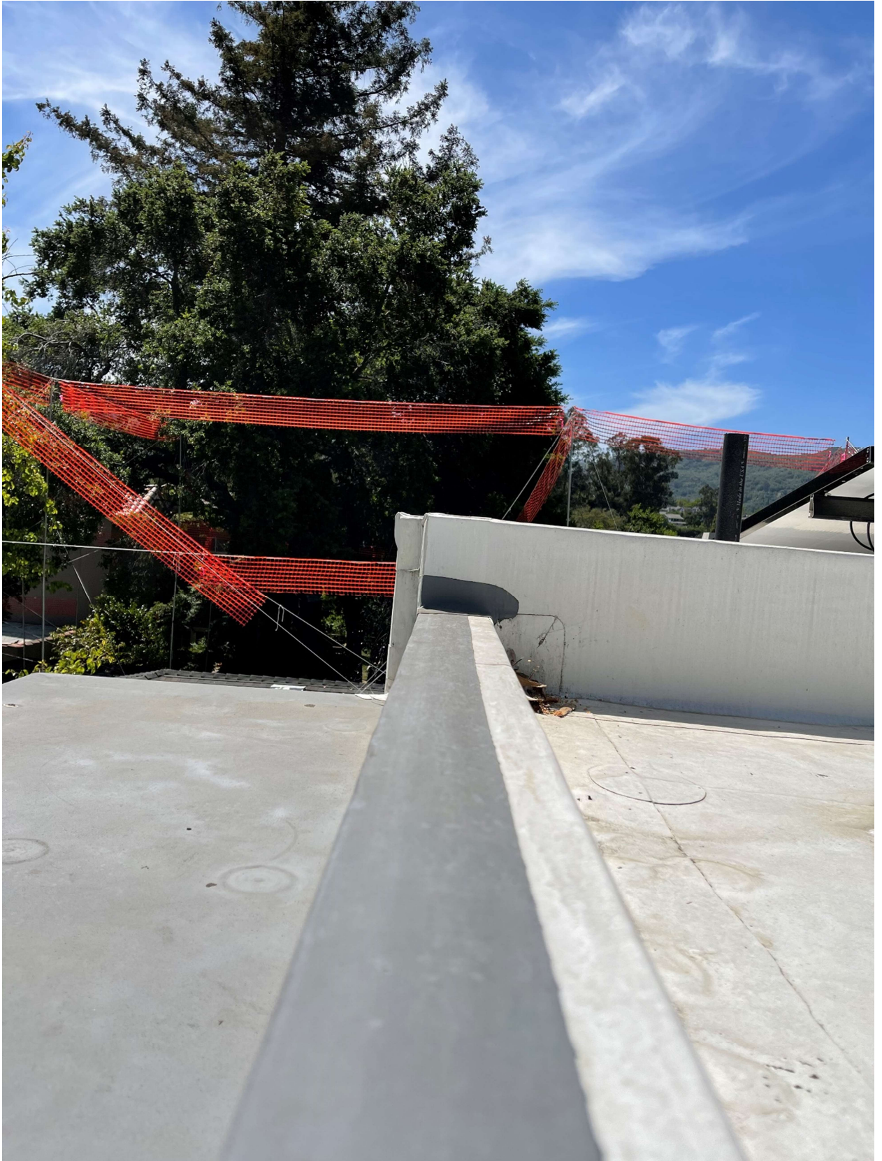
4. Rooftop View facing west (from 104 Alta Heights Ct)
