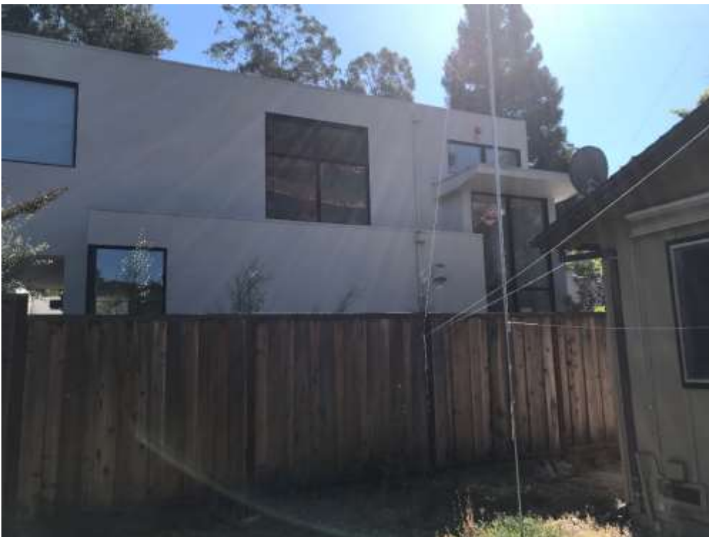
From 102 Alta Heights Court - View looking East-SouthEast at 104 AHC, the rear story pole of the proposed house is on the right. Please note that the 102 AHC is slid forward in order to preserve the mountain views for 104 AHC over the backyard of 102 AHC.
