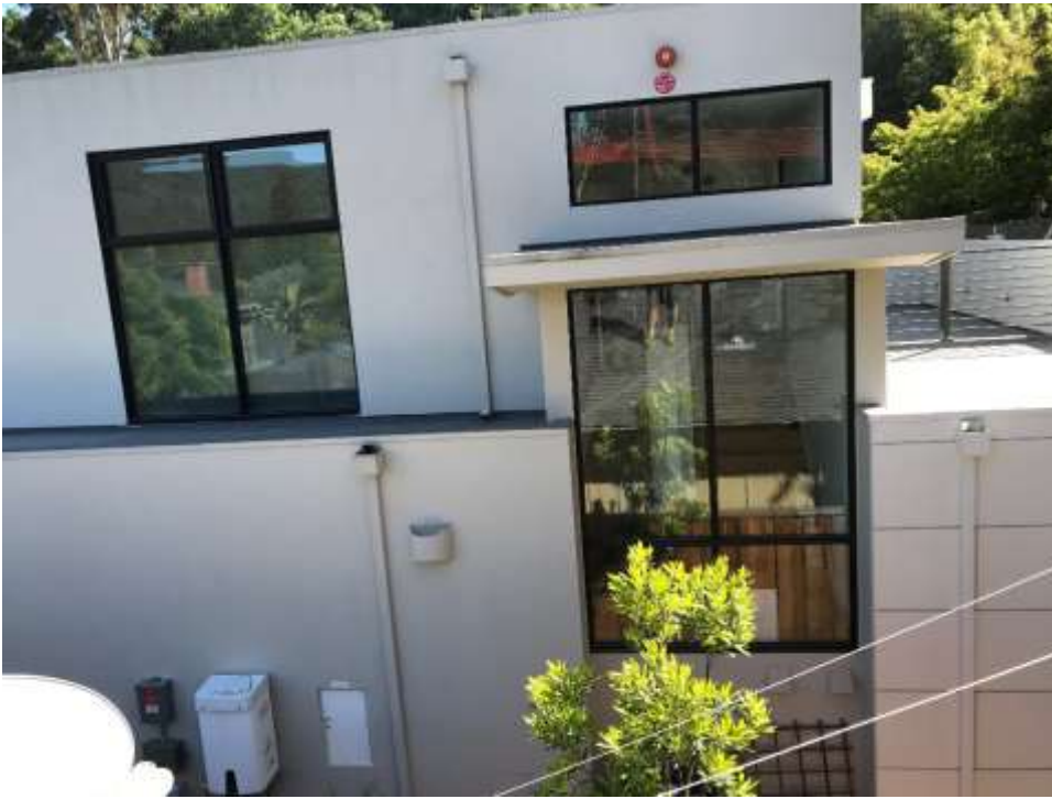
From 102 Alta Heights Court roof - View looking East at 104 AHC
