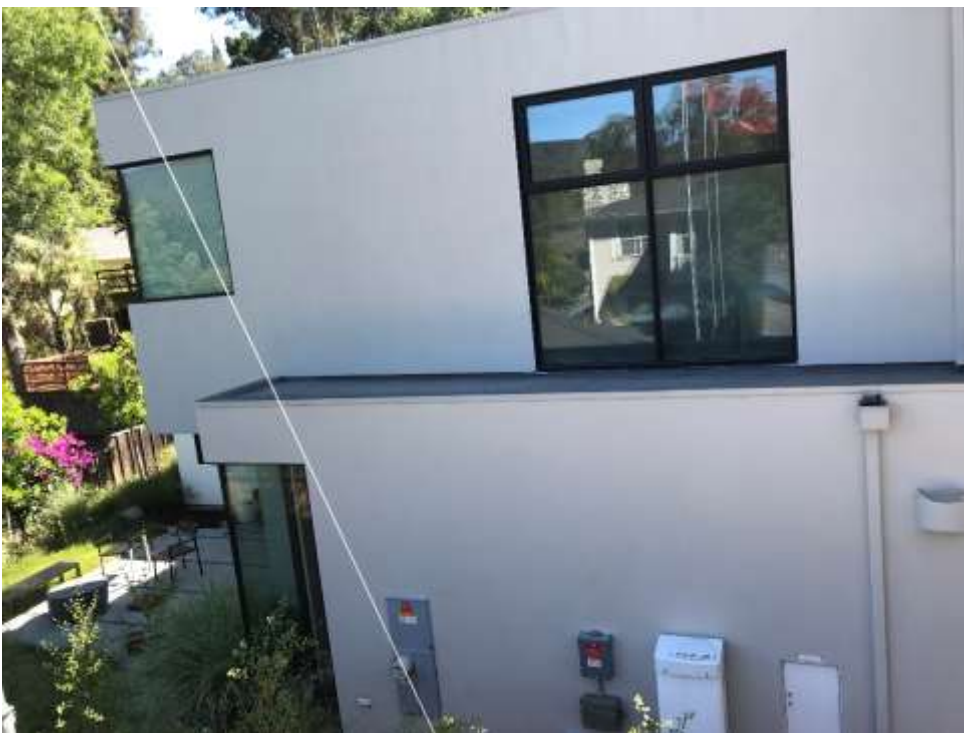
From 102 Alta Heights Court roof - View looking East-NorthEast at 104 AHC
