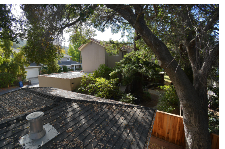
VIEW SOUTHWEST FROM ROOF
