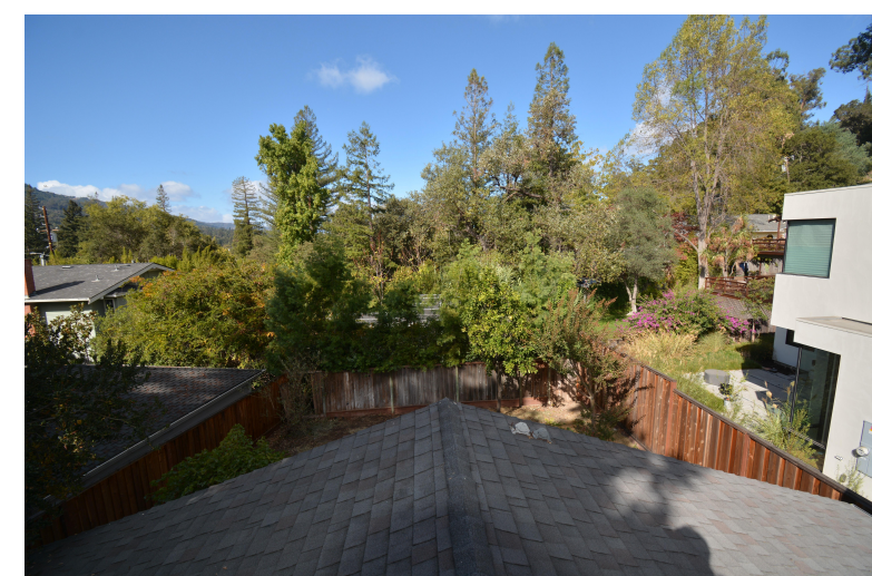
VIEW NORTH FROM ROOF
