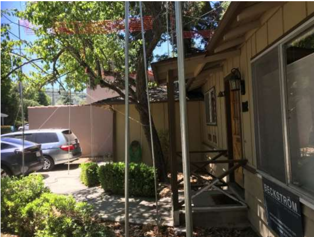
View West showing that the proposed front elevation is nearly the same as the existing house front porch. The second story pole on the left is the cantilevered front bay.
