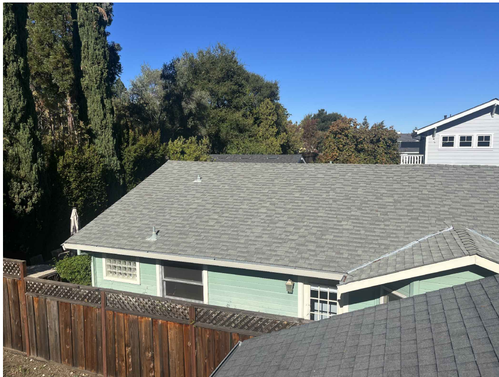
VIEW TOWARDS NORTH:
