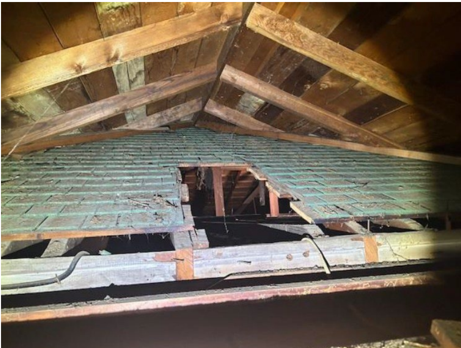
Figure 15. Detail view in attic space showing original wood shingles concealed due to rear addition, 2024. Source: Property owner.
