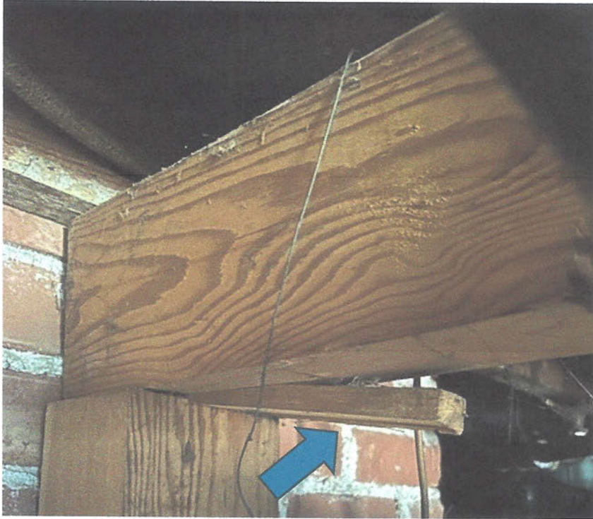
Undersized Attic Framing - 1x6 ridge beams
