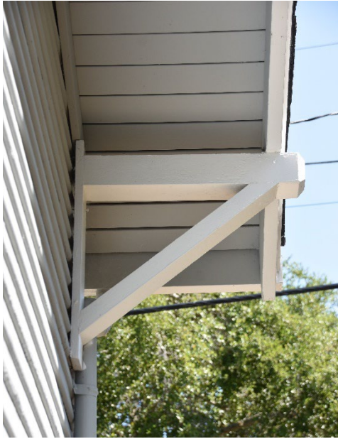
Figure 8. Applied knee brace.
