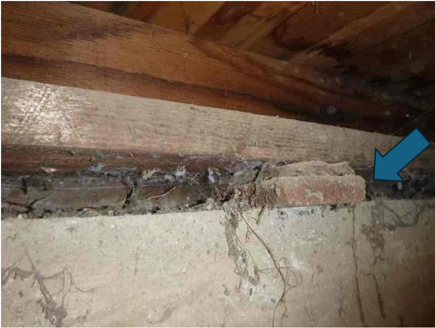
2B. Shimmed floor joists and mud sill
