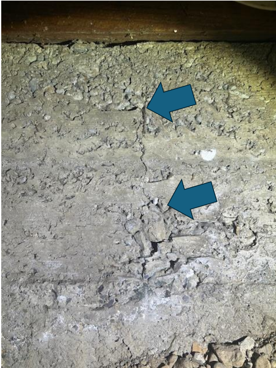
1B. Vertical cracks (front right section)
