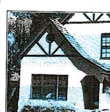
Half Timber Beams
