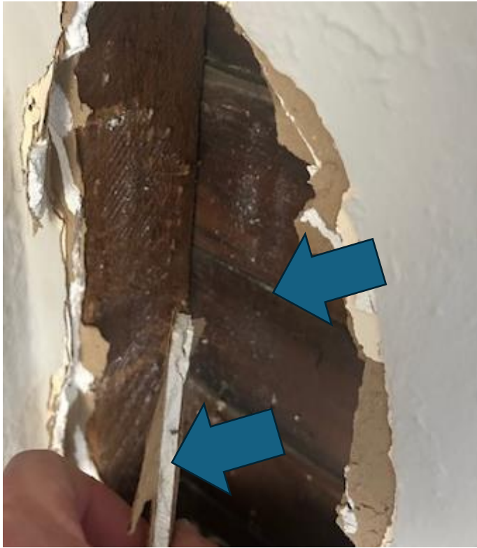
5D. Termite damage (rear door)
