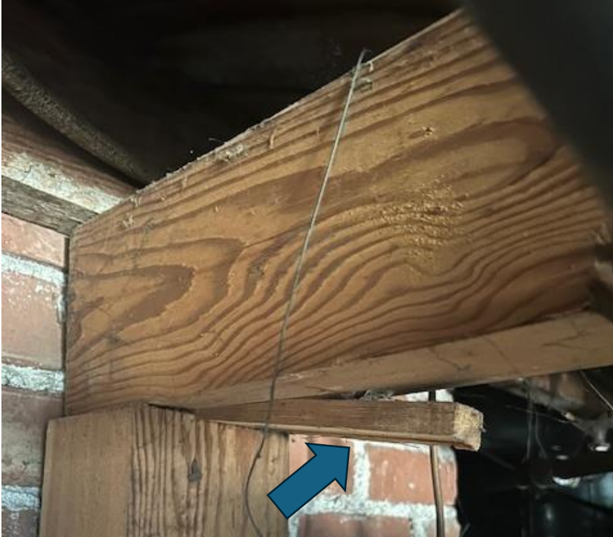
2C. Cracked 2x6 floor joists. Some spans are up to 9 feet.
