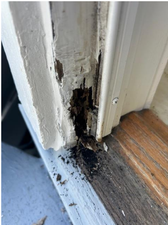
5D. Termite damage (rear door)
