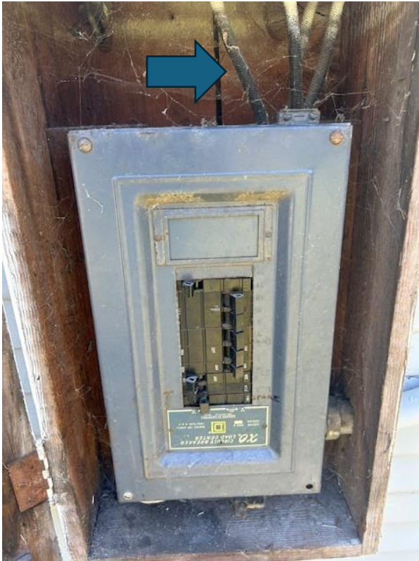
5G. Electrical Panel (unknown amps) with cloth wrapped wiring
