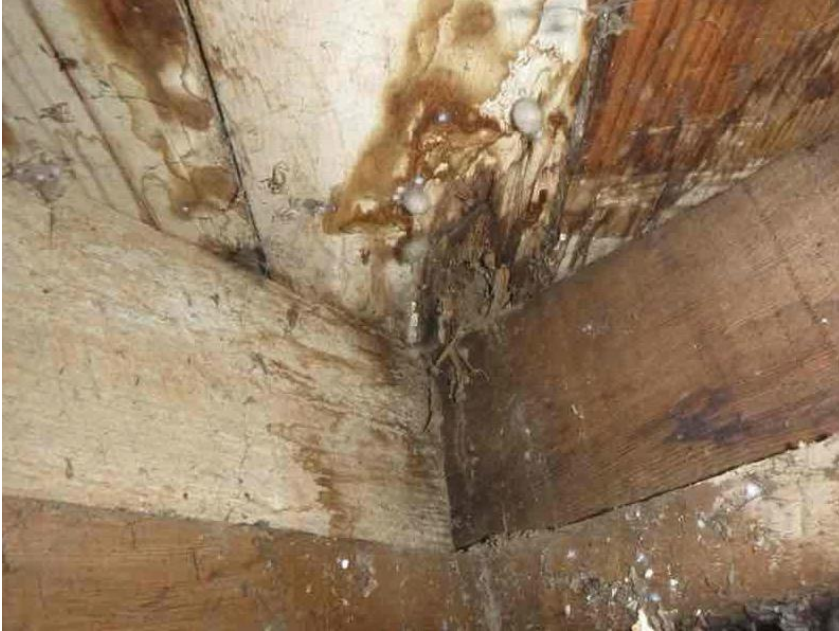
2E. Subfloor damage
