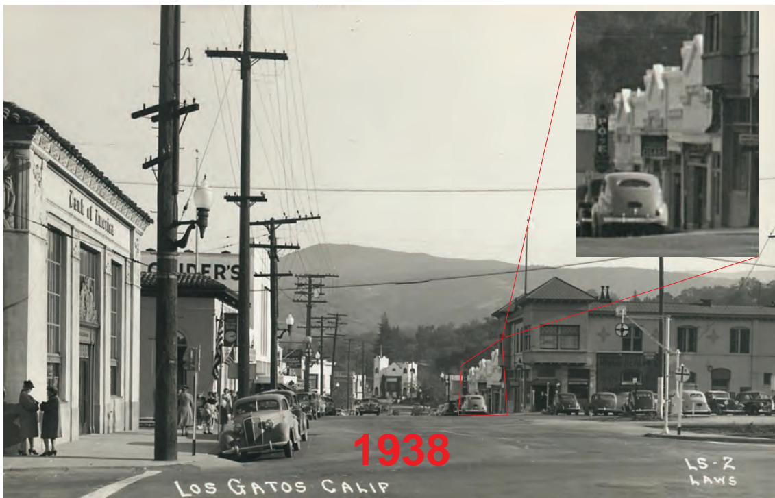
Photo clearly shows the original facades intact, including the configuration of the storefronts. The building was painted white.
