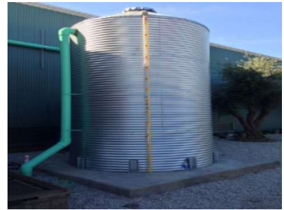
Figure 2-7 Rainwater Harvesting cistern, Environmental Innovation Center, San Jose (Source: City of San José)
