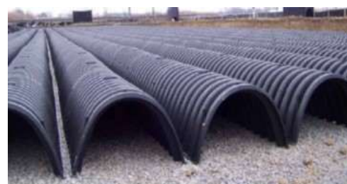
Figure 2-5 Subsurface infiltration system, (Source: Conteches.com)
