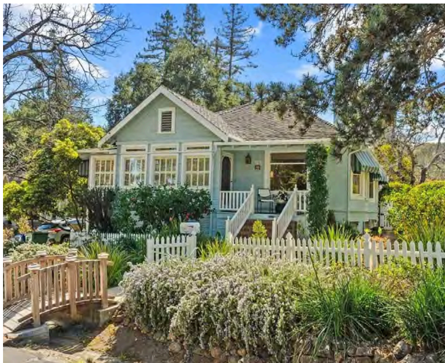
View of non-original front door location. Street view from Hernandez Ave
