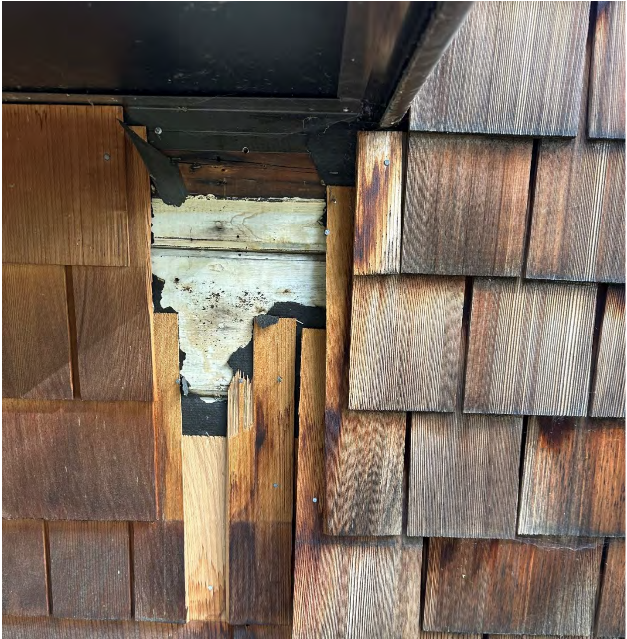
#6: South Side – Middle (original siding):
