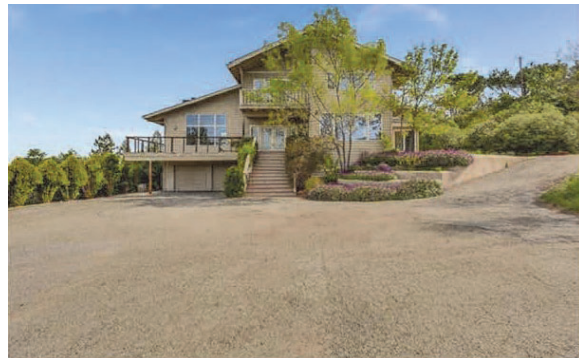
Existing House grade level view looking northeast
