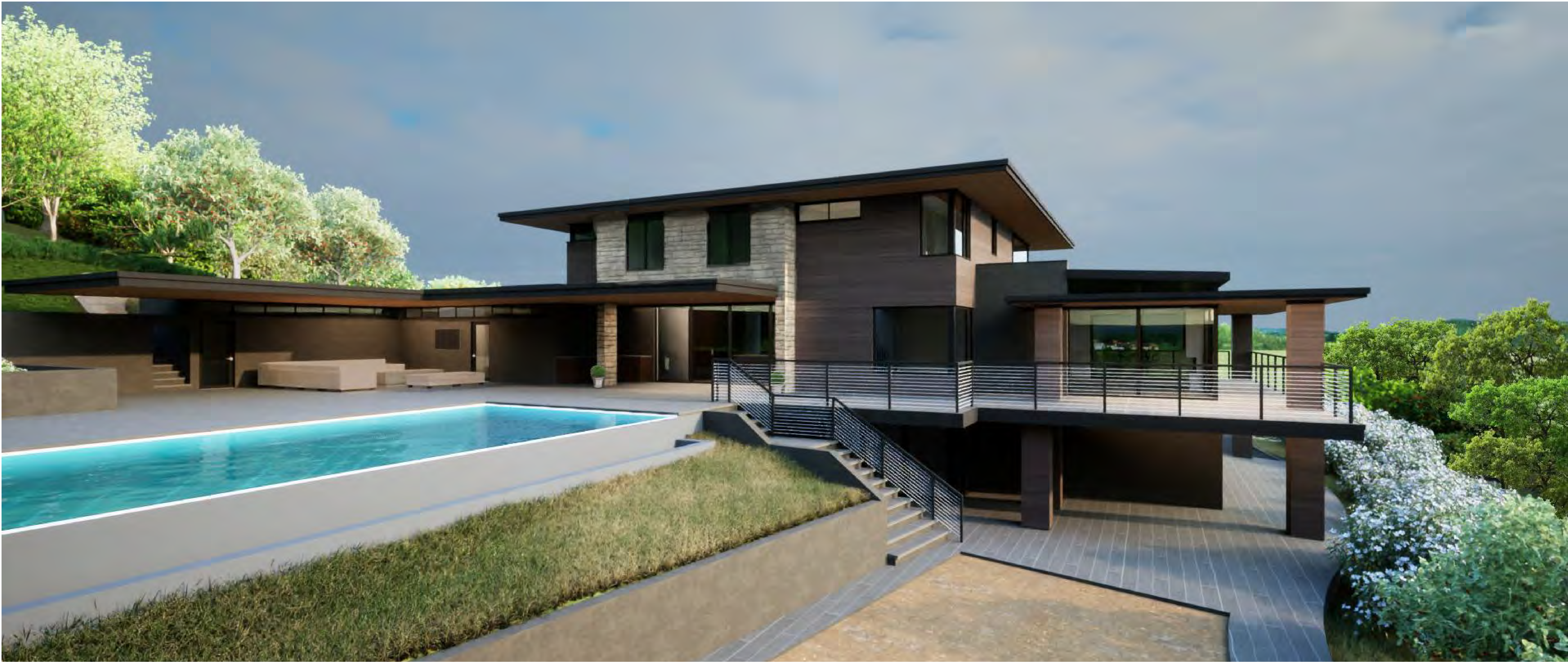
REAR NORTH VIEW-1
