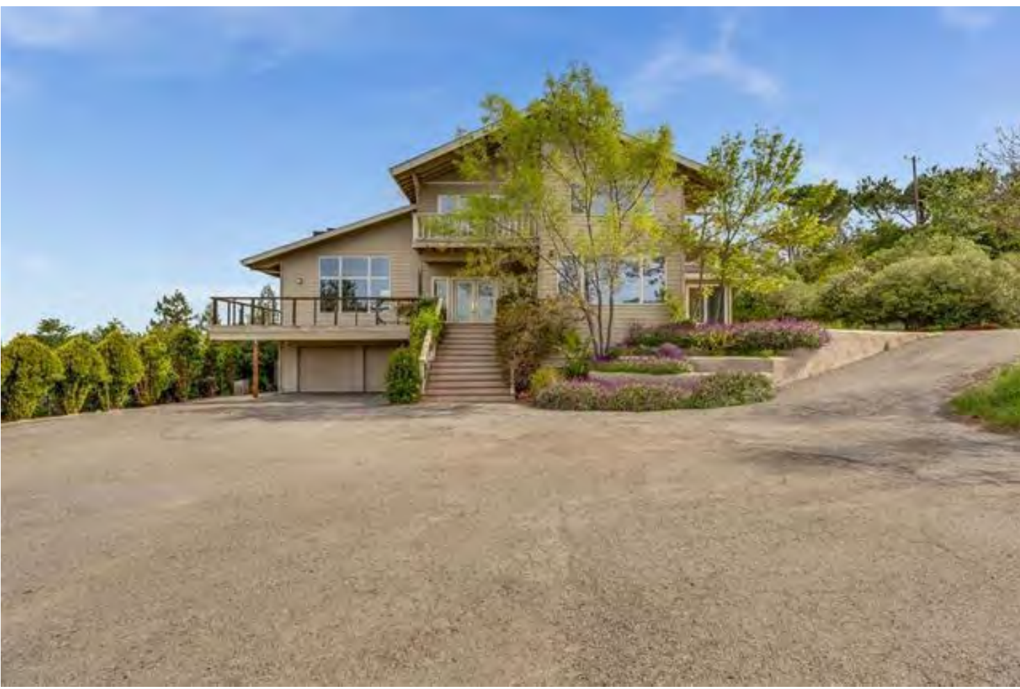
VIEW P - VIEW OF SITE LOOKING NORTHEAST
