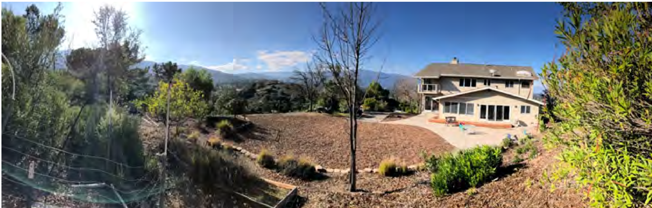
VIEW G - WIDE ANGLE VIEW OF UPPER PORTION OF BUILDING SITE - LOOKING WEST
