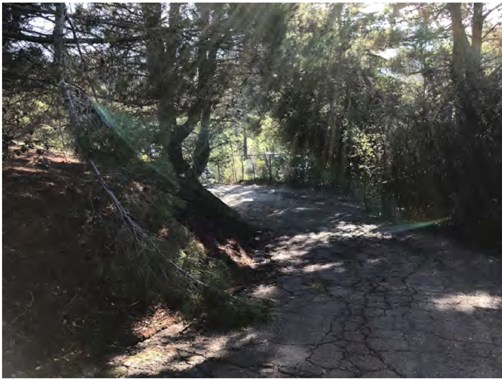
VIEW A - LOWER DRIVEWAY - LOOKING SOUTH
