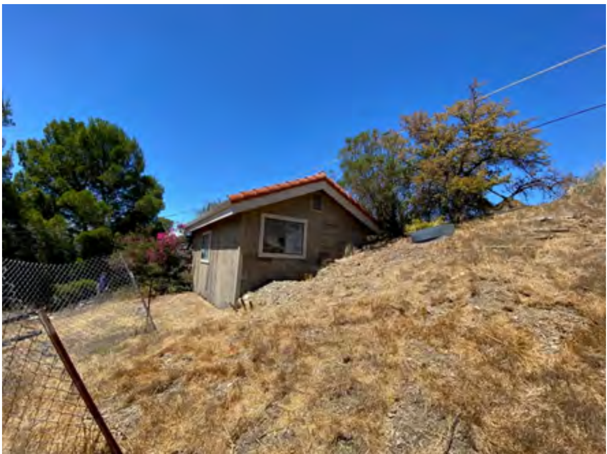
VIEW N - SHED - HILLSIDE BELOW BUILDING SITE - LOOKING NORTH
