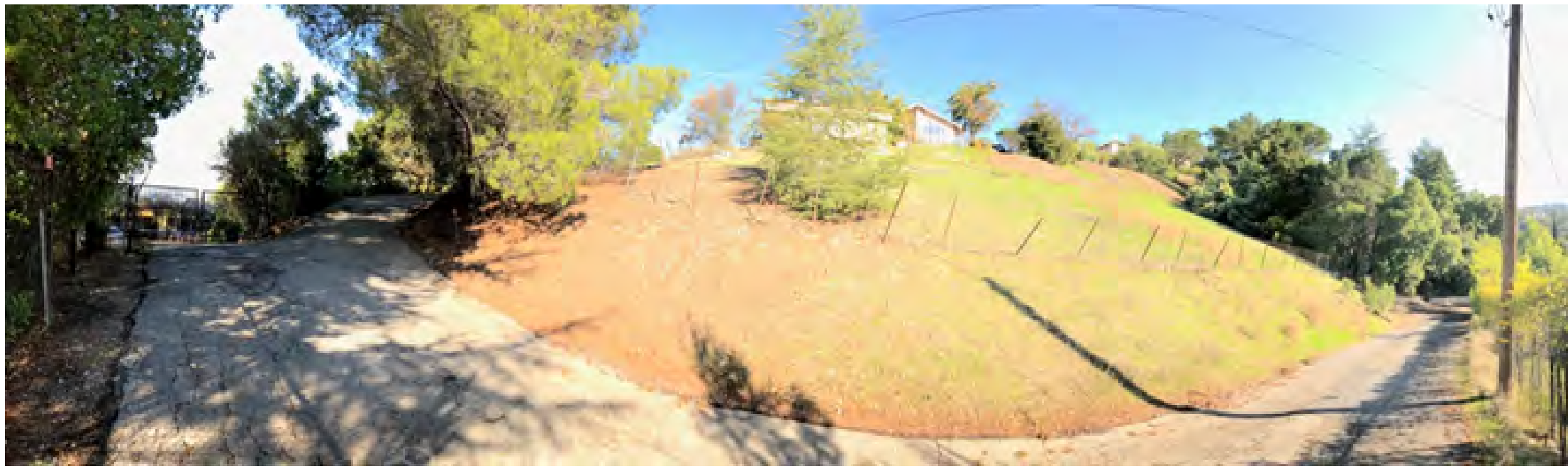
VIEW C - WIDE ANGLE VIEW OF LOWER DRIVEWAY - LOOKING SOUTHEAST
