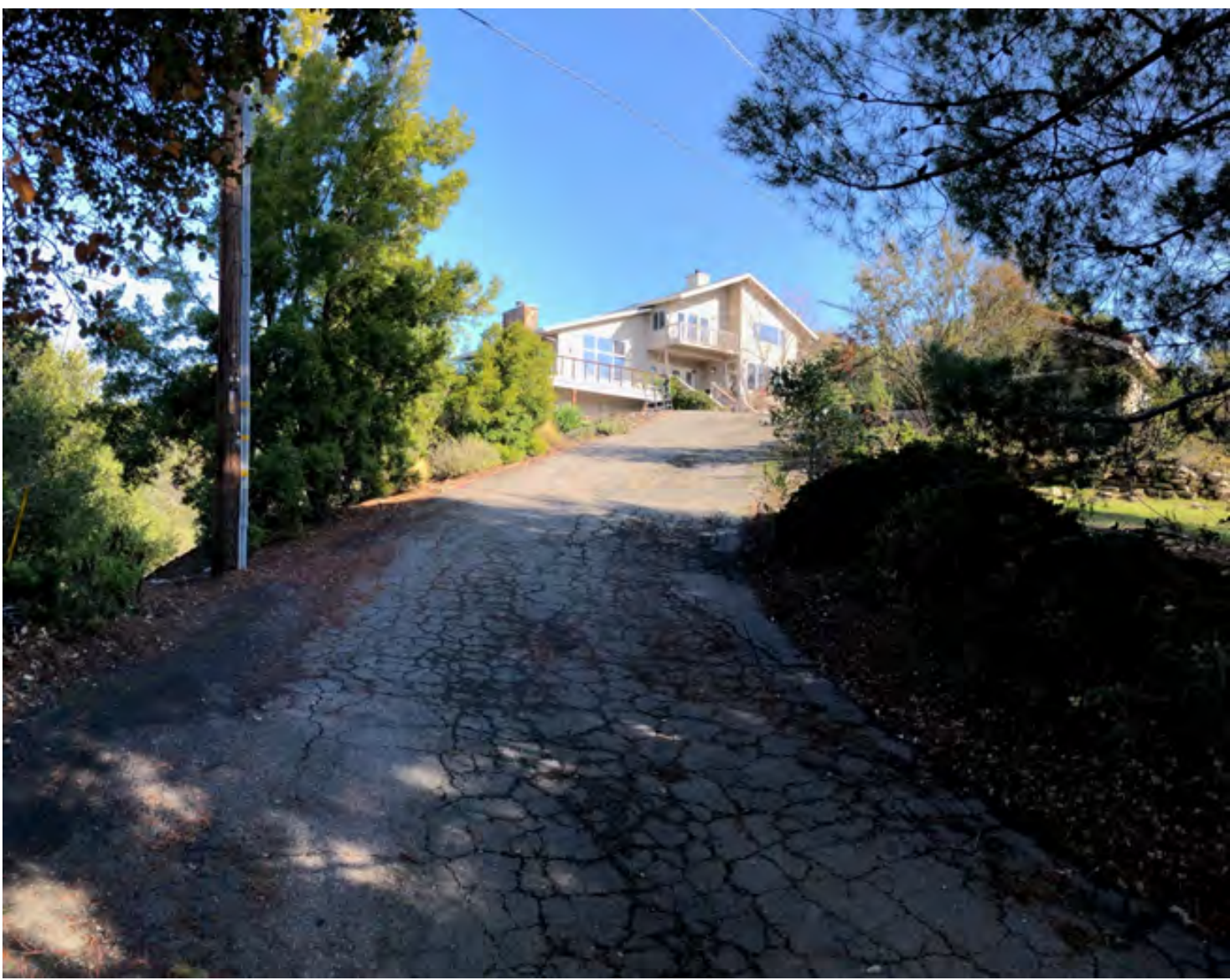
VIEW L - LOWER DRIVEWAY TOWARD BUILDING SITE - LOOKING NORTHEAST
