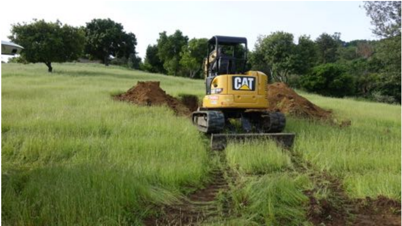
Photo 3: View of backhoe excavating Test Pit 1.
