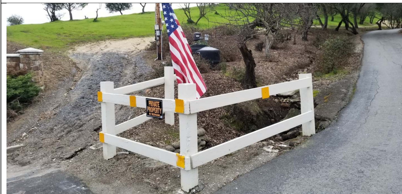
13. Town Barricade at Storm Headwall
