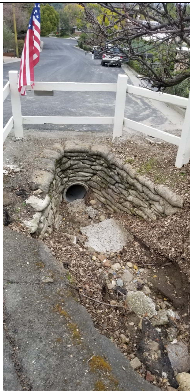
3. Drainage Headwall
