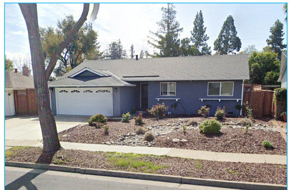
Nearby house to right
