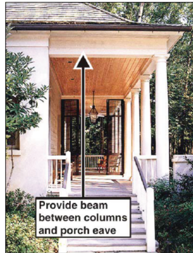
Porch beam example with good depth and details
