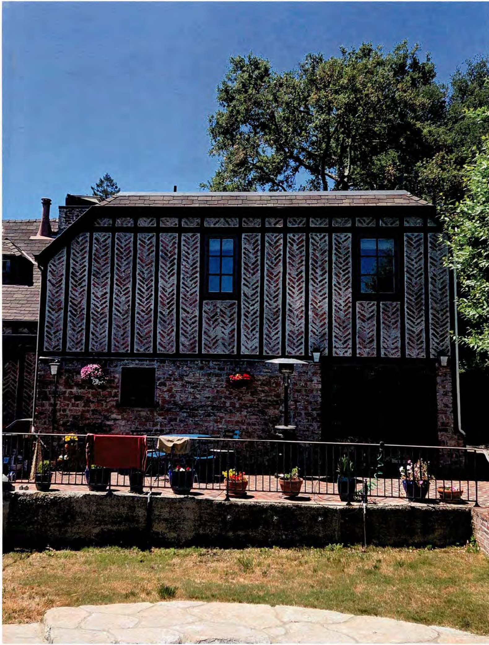
SUBJECT REAR WALL #1 (NORTHEAST)
