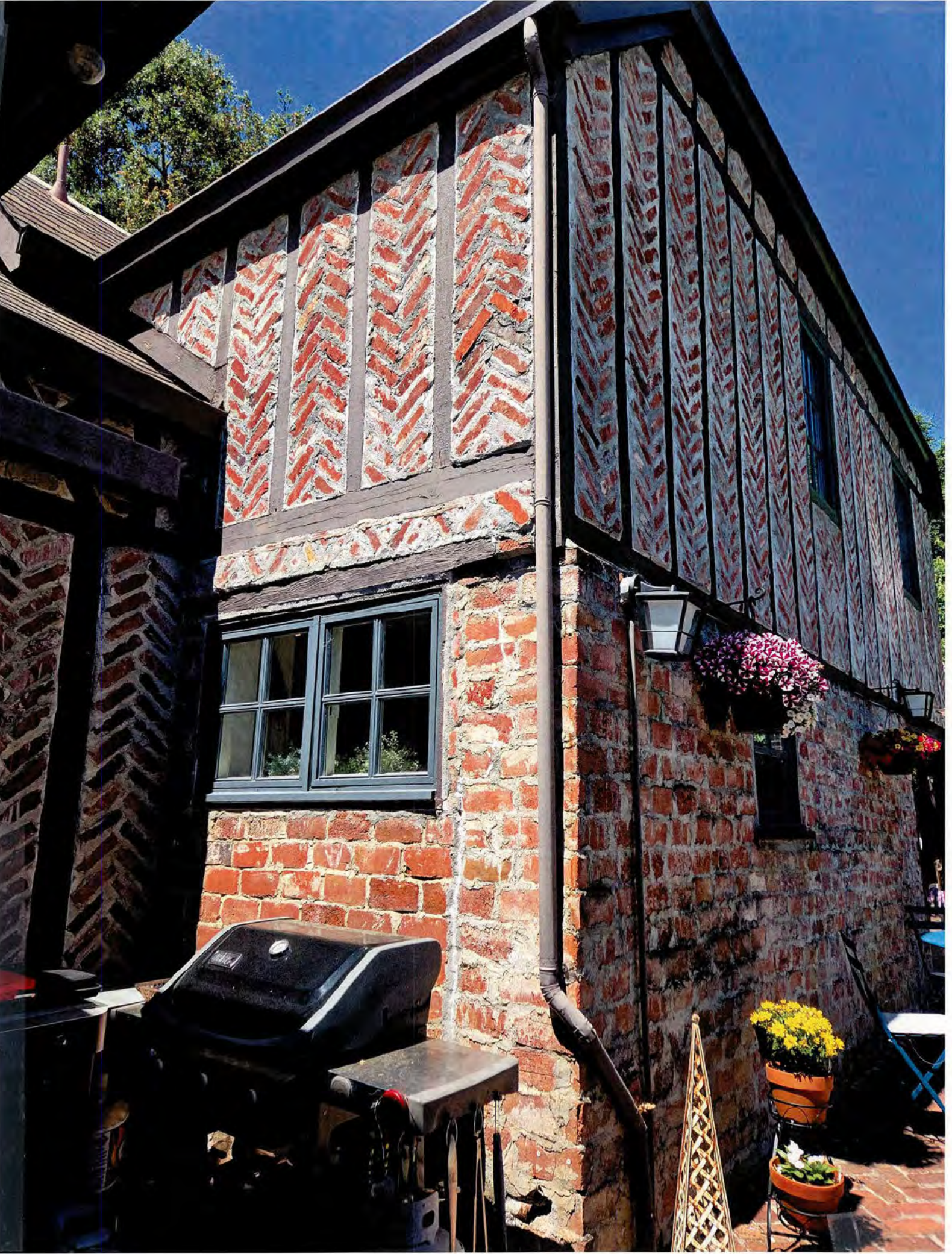
KITCHEN WINDOW TO REMAIN (SOUTHEAST)
