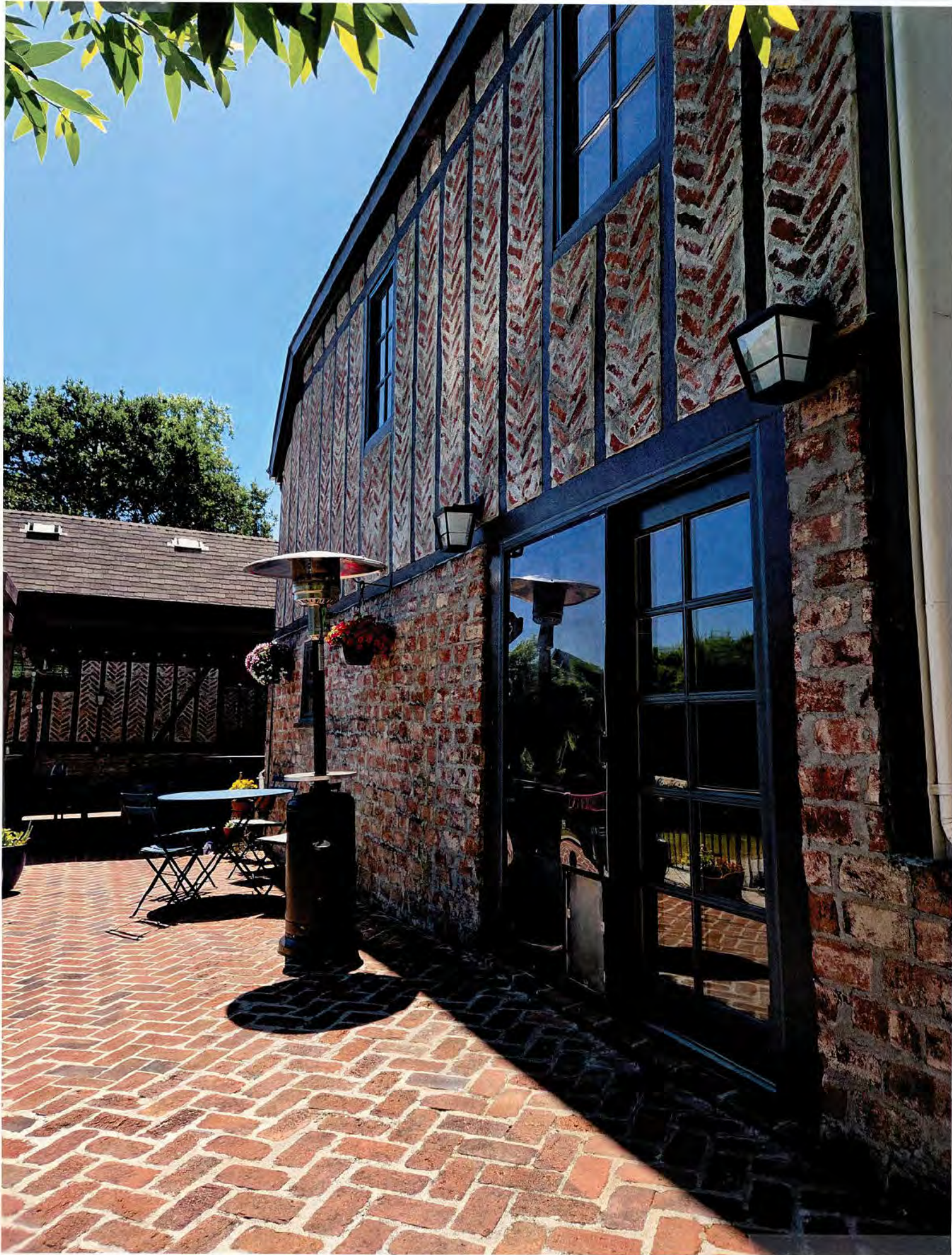
SUBJECT REAR WALL #2 (NORTHEAST)
