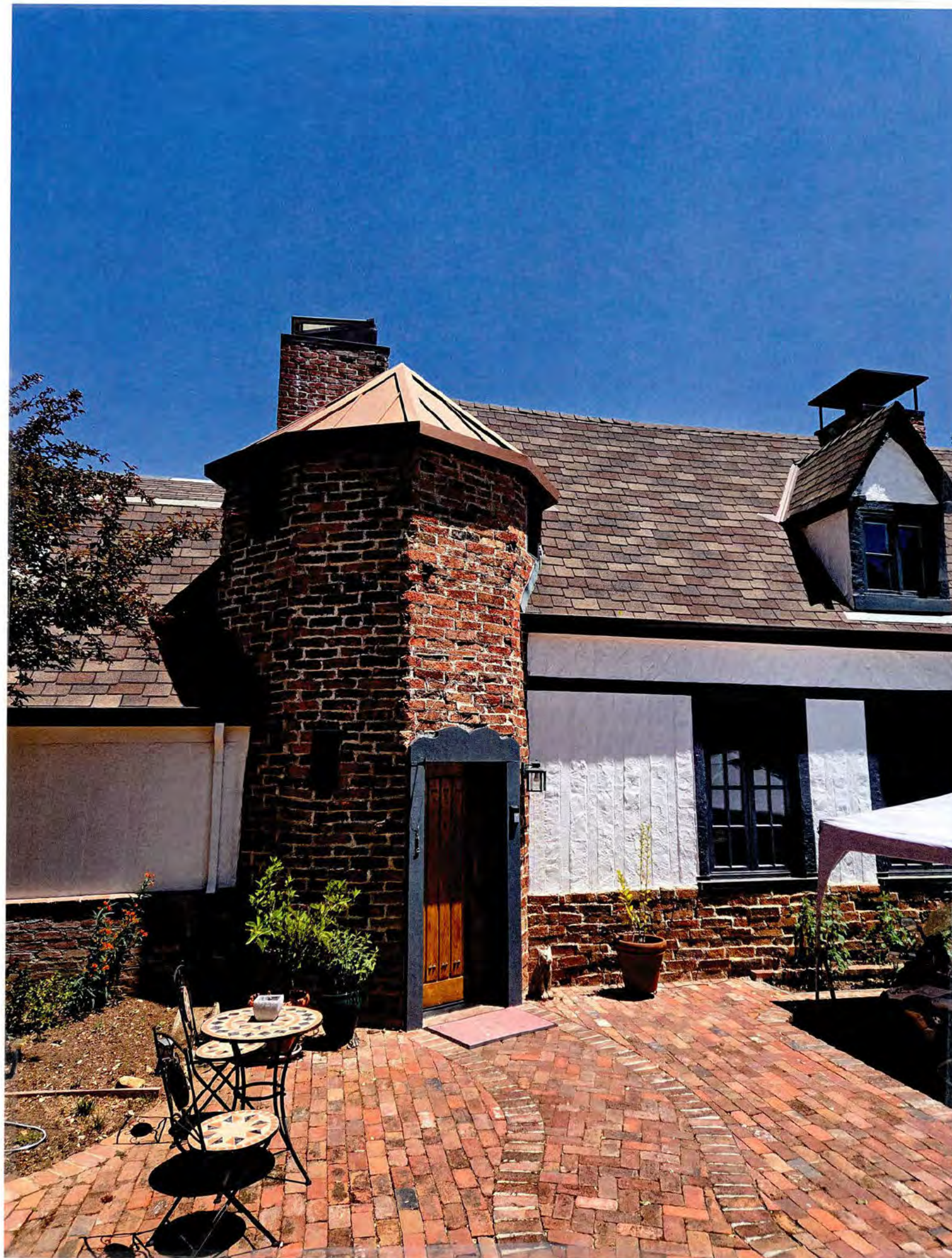
EXISTING FRONT ENTRY (SOUTHWEST)
