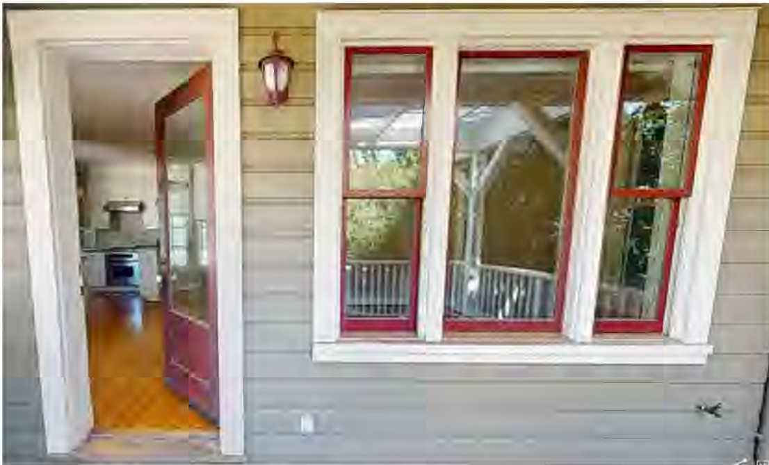
EXISTING PAINTED WOOD DOOR AND WINDOWS. WINDOW TRIM 2X ROUGH SAWN WOOD W/ STOOL AND APRON
