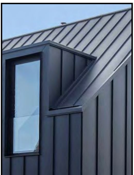
4 STANDING SEAM METAL ROOF
