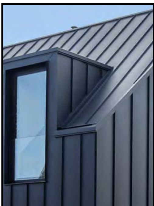
4 STANDING SEAM METAL ROOF
