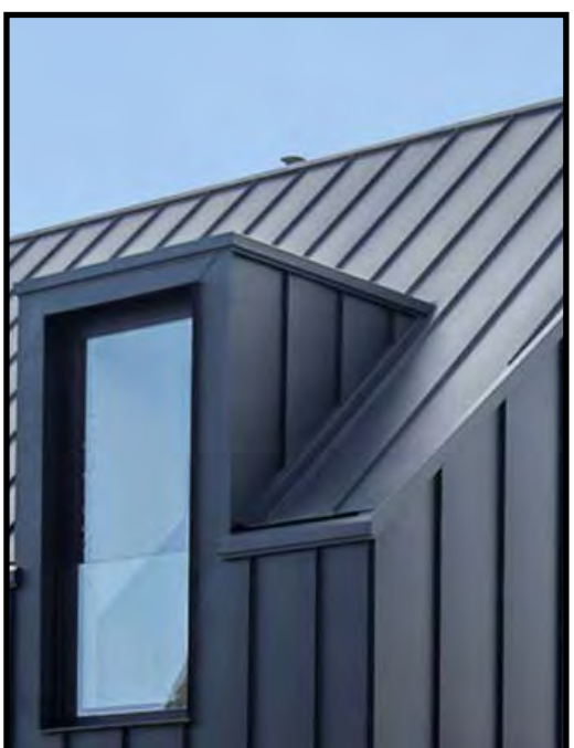
4 STANDING SEAM METAL ROOF
