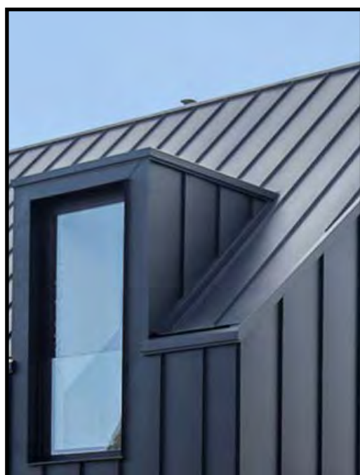
4 STANDING SEAM METAL ROOF
