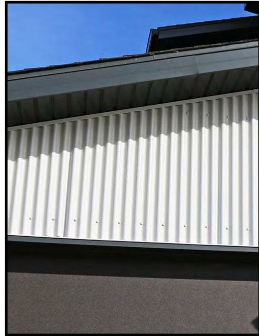
6 VERTICAL CORRUGATED METAL SIDING
