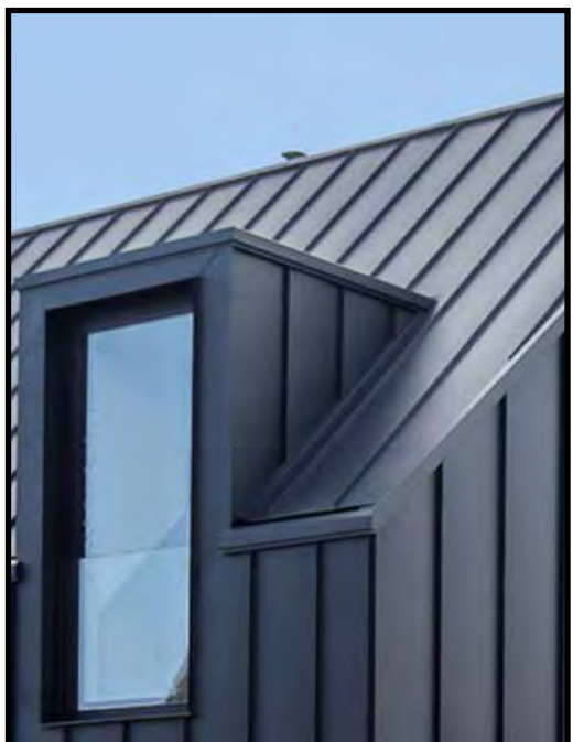
4 STANDING SEAM METAL ROOF
