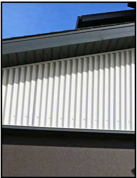
6 VERTICAL CORRUGATED METAL SIDING
