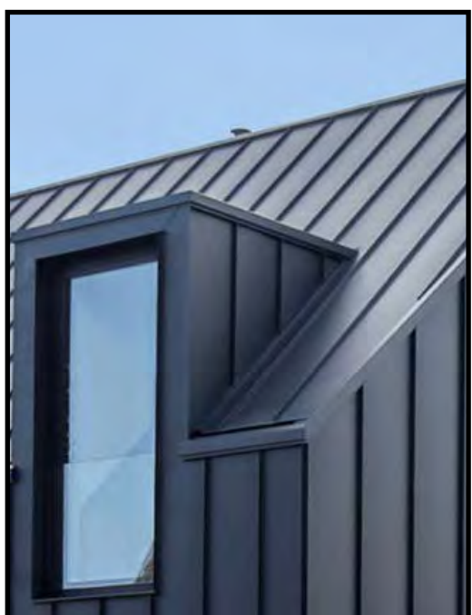
4 STANDING SEAM METAL ROOF
