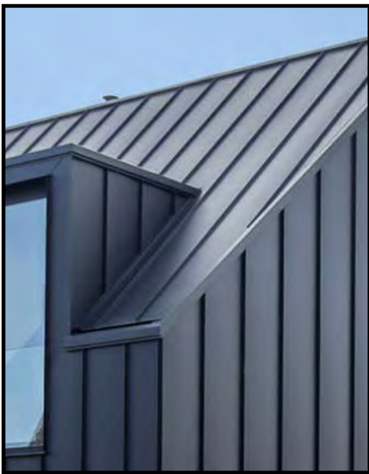
7 STANDING SEAM METAL ROOF
