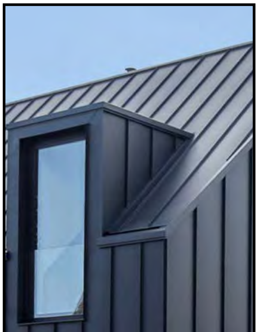
4 STANDING SEAM METAL ROOF
