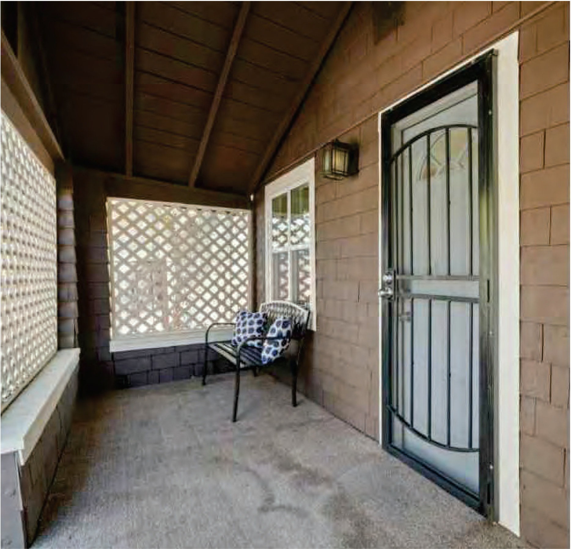
6. ENTRY FOYER (PORCH)
