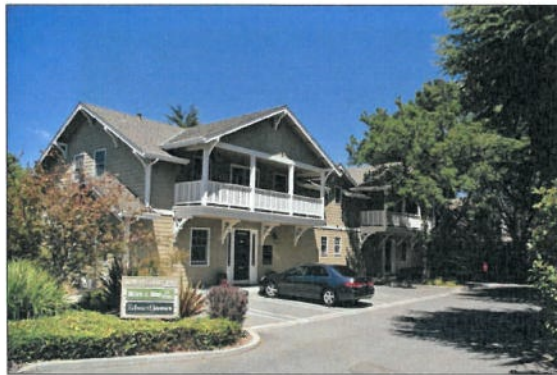
Immediately adjacent office building on Los Gatos Blvd.
