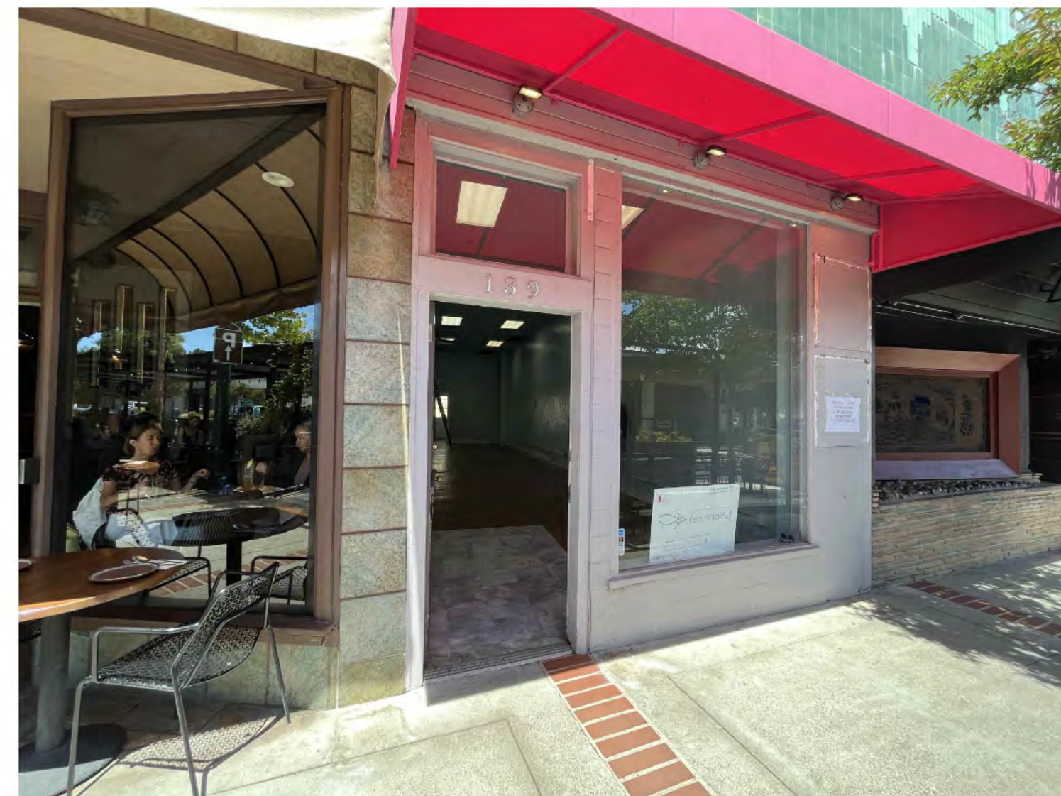
139 N SANTA CRUZ AVE: EXISTING EXTERIOR
