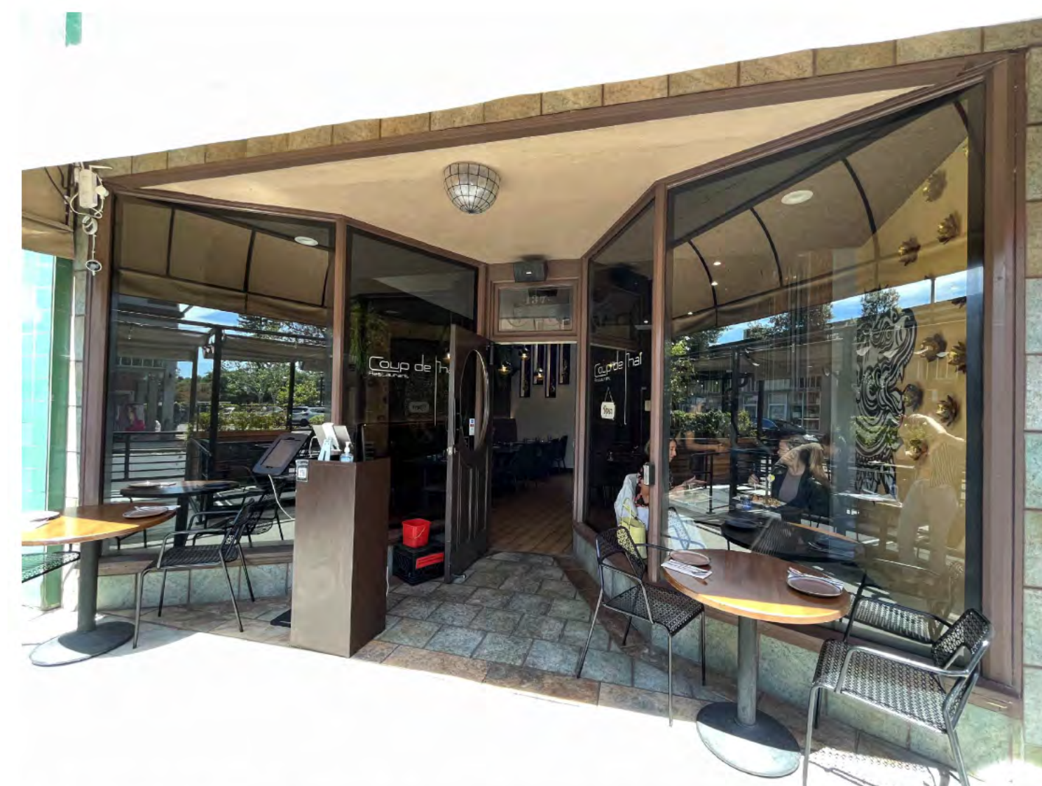
137 N SANTA CRUZ AVE: EXISTING EXTERIOR
