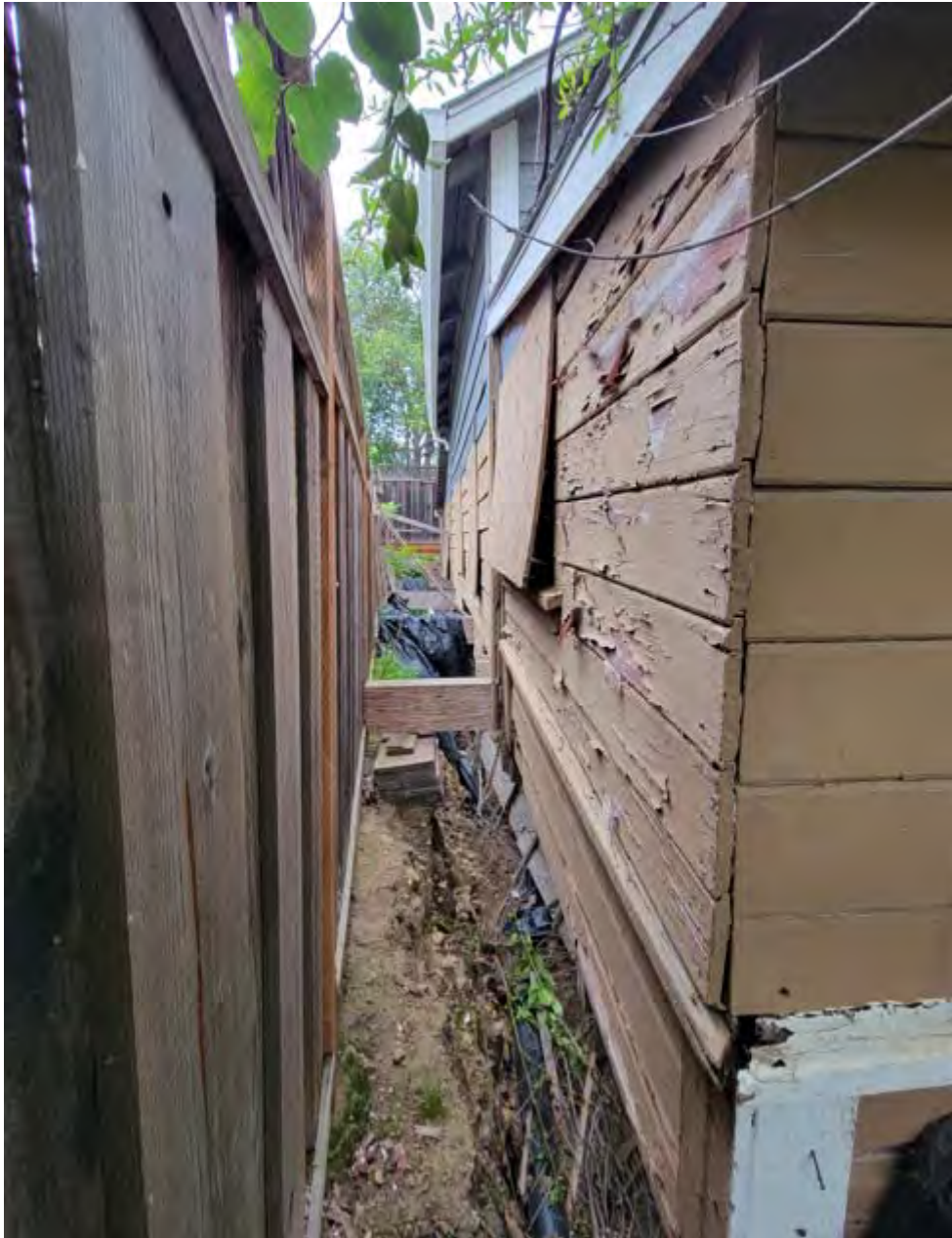
Exterior View – West Side
