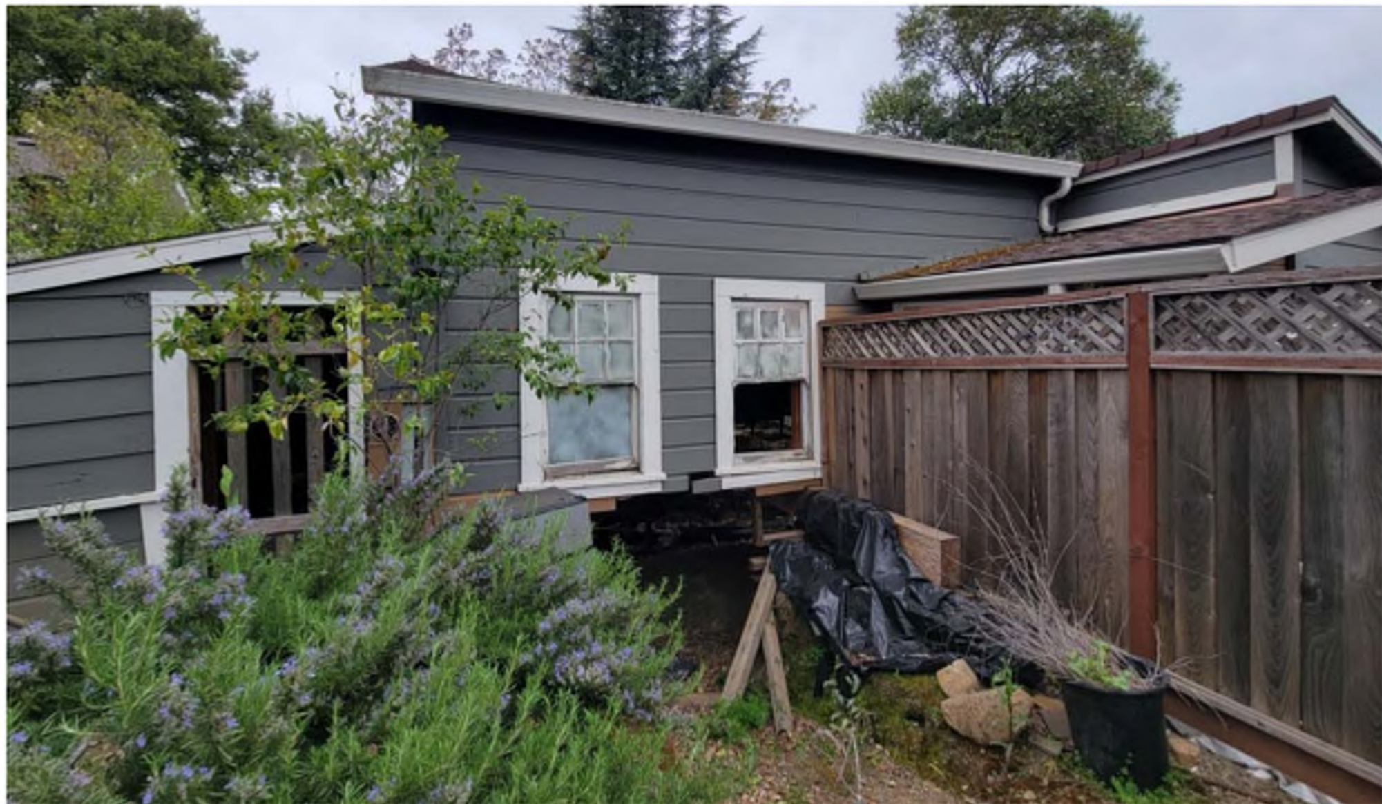
Exterior View East Side
