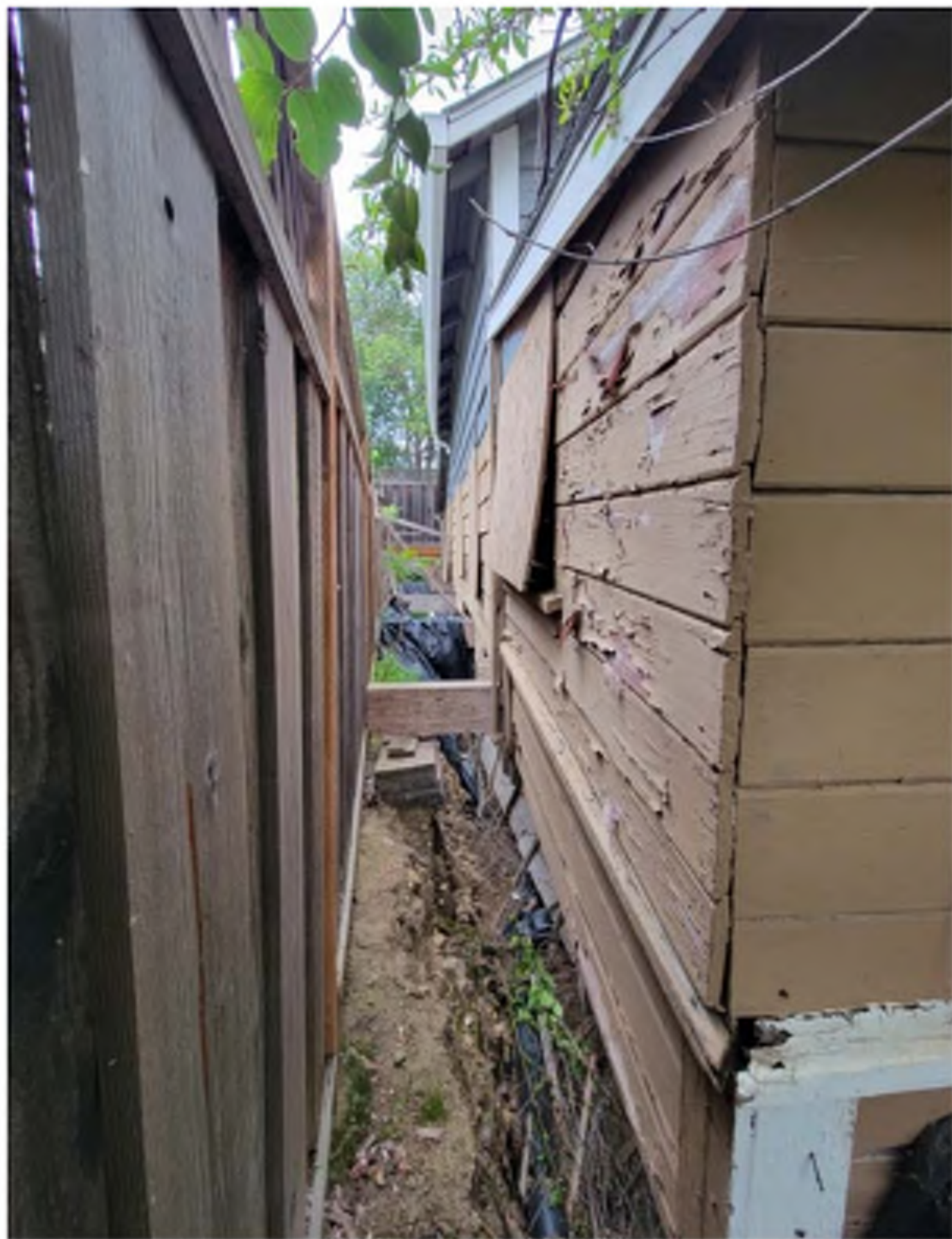
Exterior View – West Side
