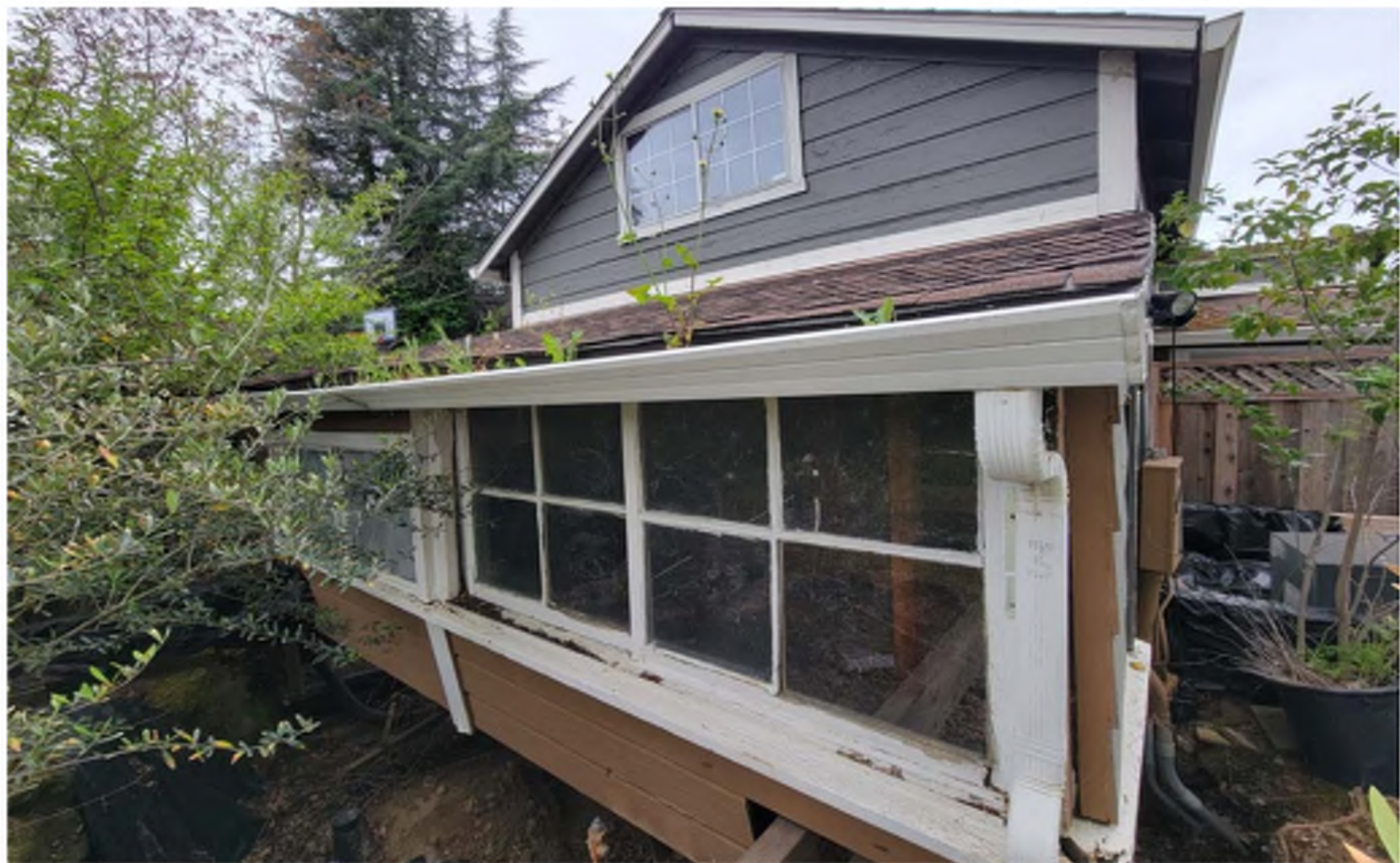
Exterior View - South Side
