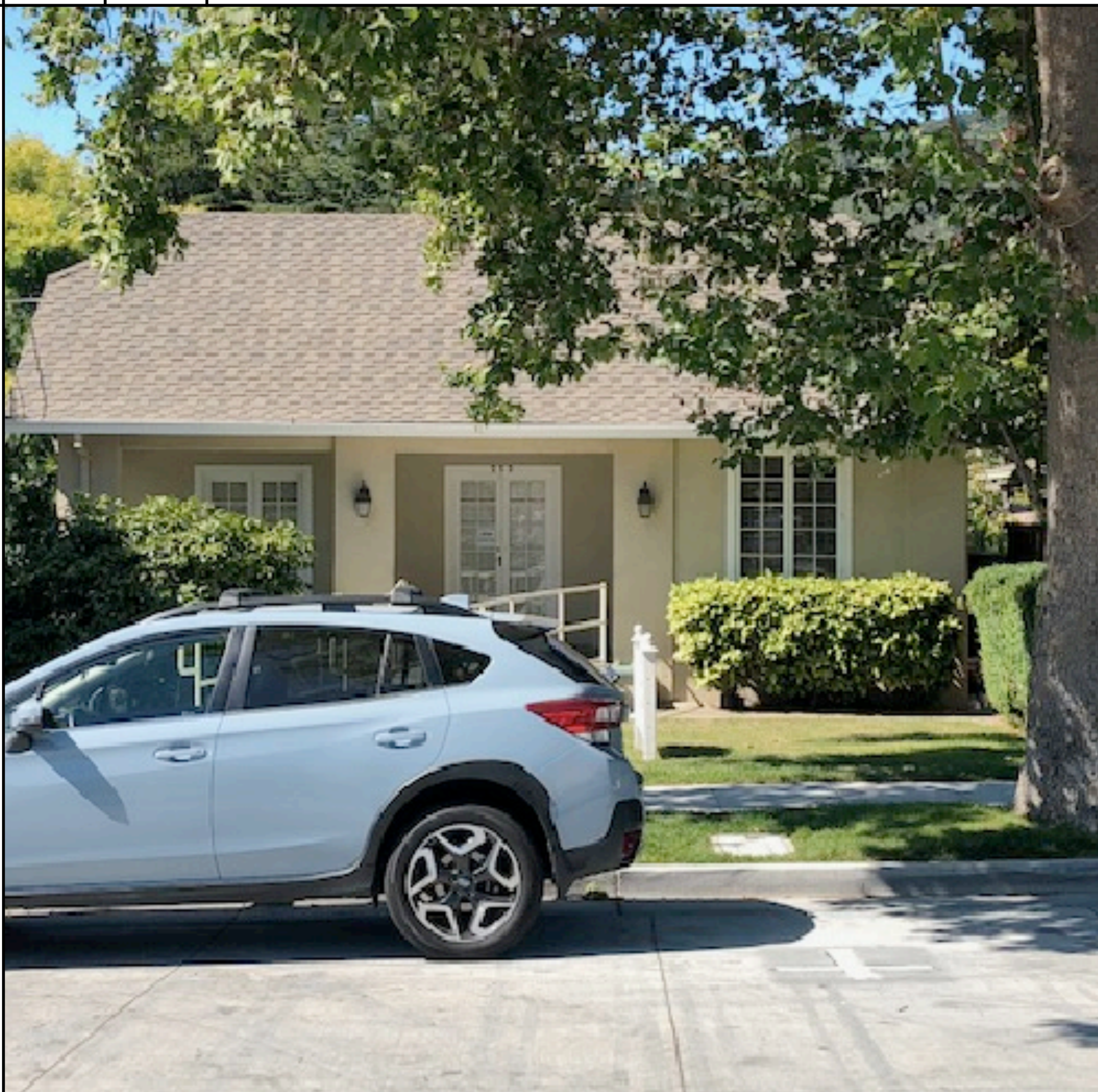
D NTS EXISTING HOUSE ACROSS STREET - 253 ALMENDRA AVE.
