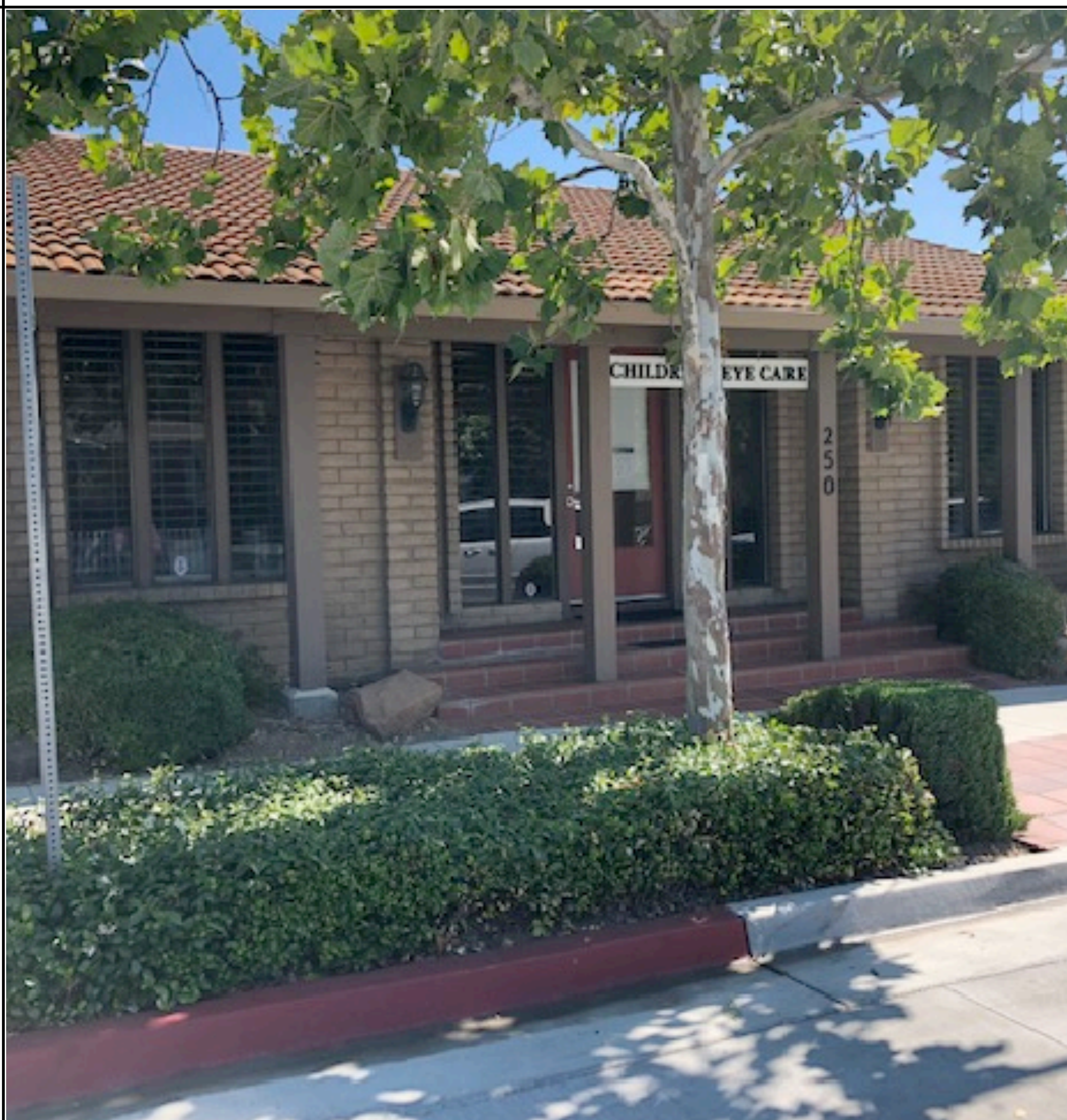
A NTS EXISTING ADJACENT MED. OFFICE - 250 ALMENRDA AVE.
