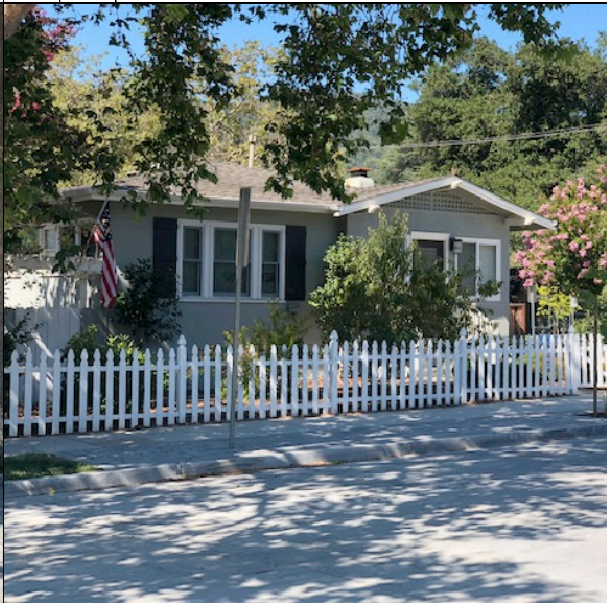
E NTS EXISTING HOUSE ACROSS STREET - 259 ALMENDRA AVE.
