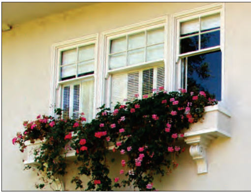
True divided lite windows are encouraged when appropriate to the original structure
