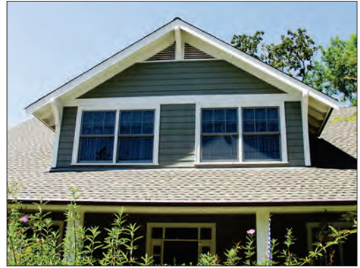
Heavy profile fireproof composition shingles may be used as a replacement for wood single and wood shake roofs
