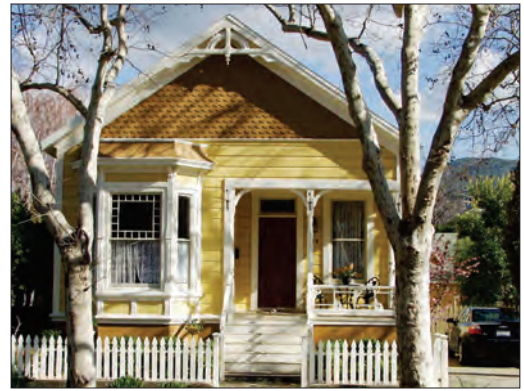
Match bay windows to the architectural style of the house
