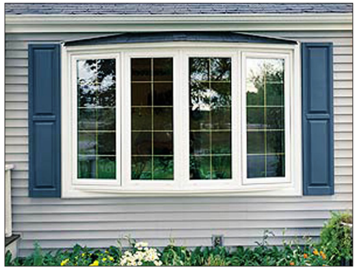
Some window styles, such as this bow bay window, would have very limited applicability for use on a historic resource structure
