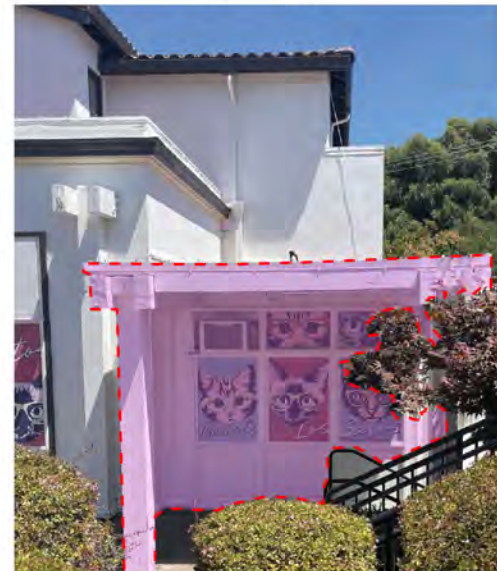
SCOPE OF WORK AREA: HIGHLIGHT OF UNPERMITTED ADDITION TO BE REMOVED
