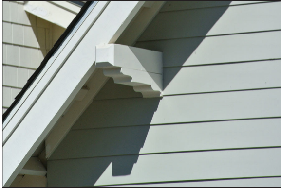
Gable end supports
