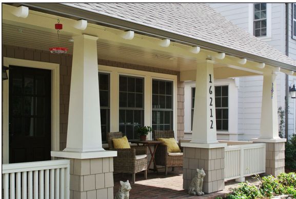
Porch beams and columns
