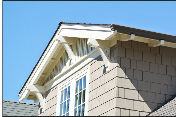
Gable end supports
