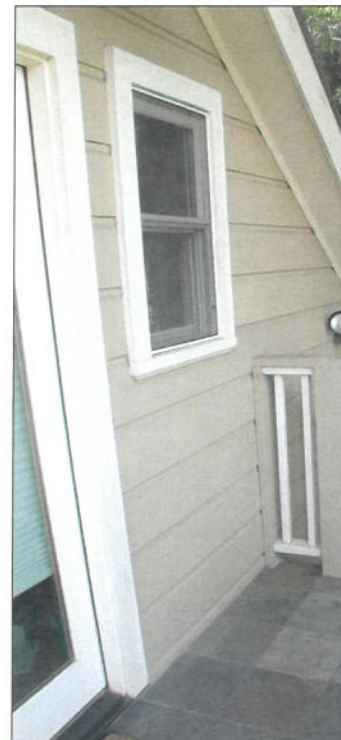
EXISTING WINDOW PHOTO
