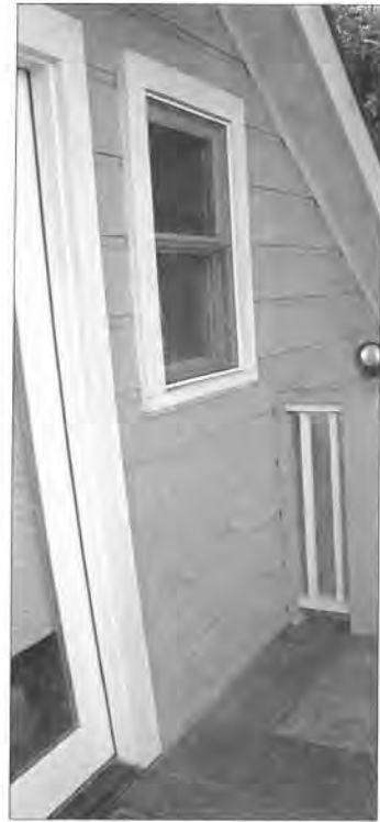
EXISTING WINDOW PHOTO
