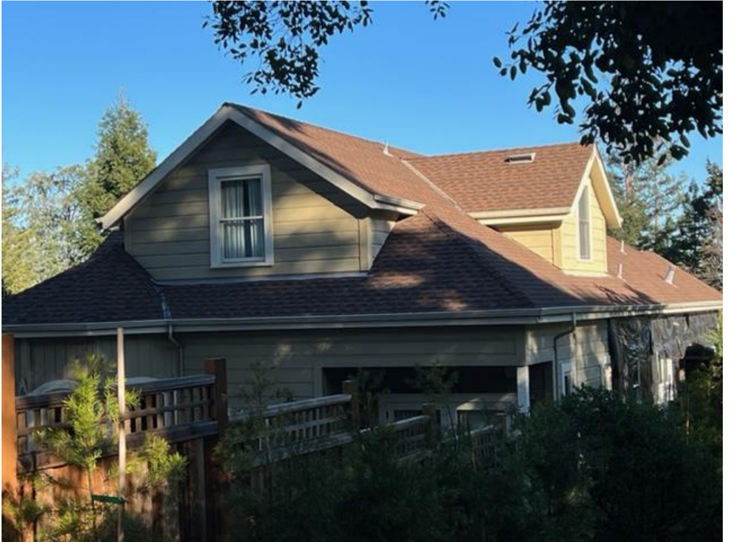
8. Southwestern Elevation (from Wissahickon) view of three-gabled second-story addition:
