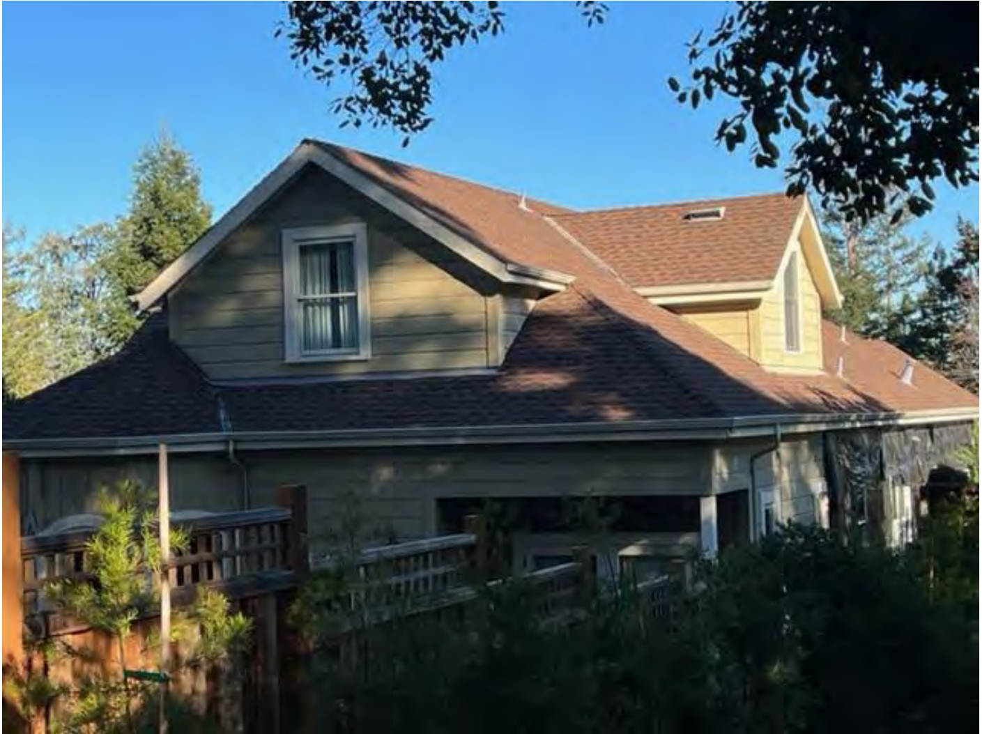
5. Southwestern Elevation (from Wissahickon) view of three-gabled second-story addition:
